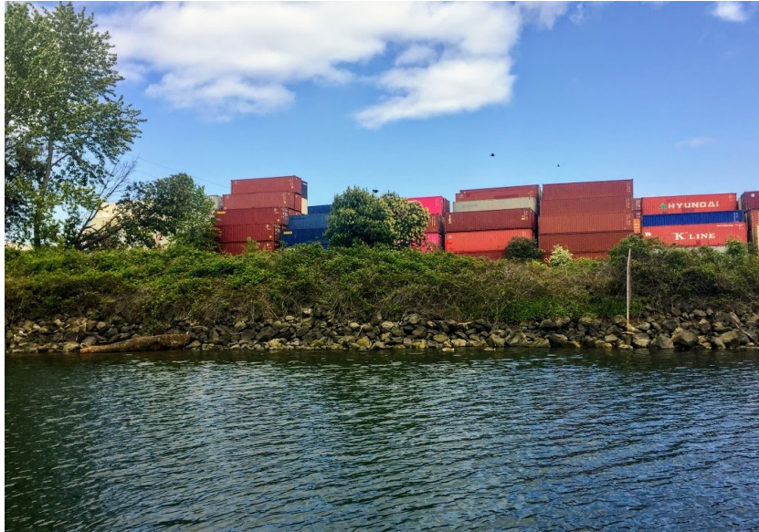
Photo: typical riprap armoring in the Duwamish River at high tide, at Terminal 108.
