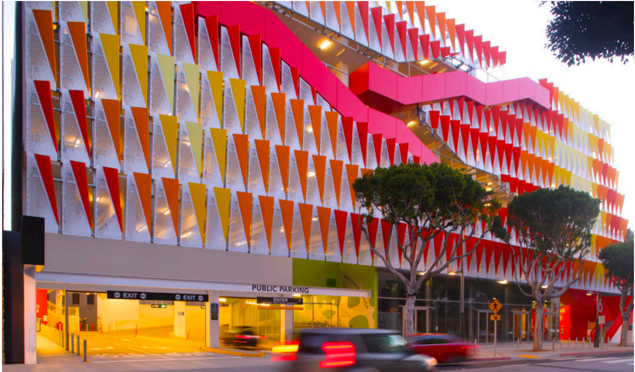
Figure 39. City of Santa Monica Public Parking Structure #6, an example of how a parking structure can contribute to its context. Structure #6 has bright, airy interiors, is LEED Gold-certified, has retail, and a farmer's market. Source: Behnisch Architekten
