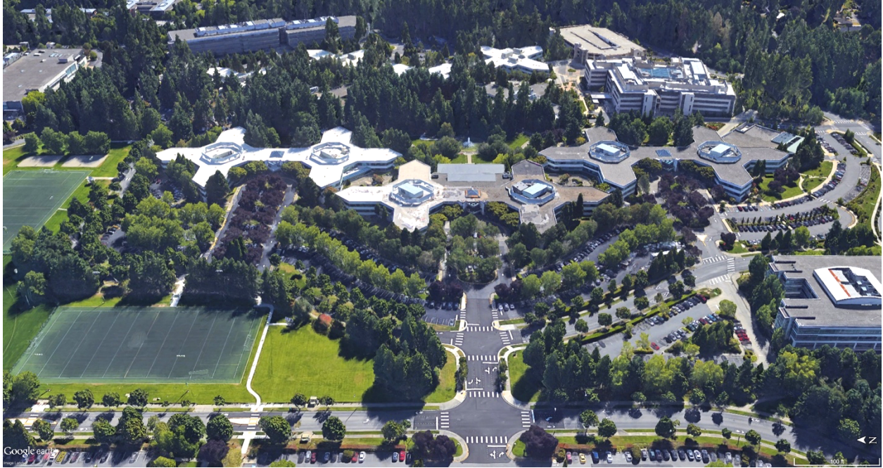
Figure 24. 'X' Buildings. 157th Ave NE/Microsoft Way at bottom. Source: Google Earth.
