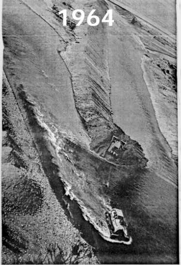
MOVING A RIVER — A bulldozer crosses the old channel after cutting through the last of gravel Thursday to allow the Elwha River to turn into a new channel at its mouth. A new bed for the river was dug after it had cut its way westward to a point where it endangered several residences at The Place near the confluence of the Elwha and the Strait of Juan de Fuca. The Strait is in top of picture. (Evening News Photo.) 7/24/64 15-84 (2)
