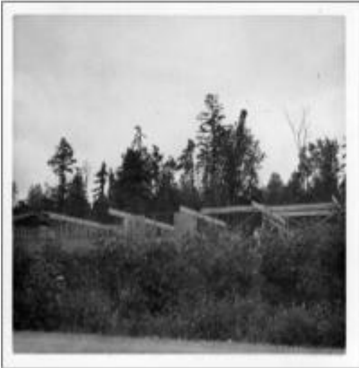
Figure 15: Wenberg House under construction, 1962. Source: Louise Bruse Wenberg Luce private collection.
