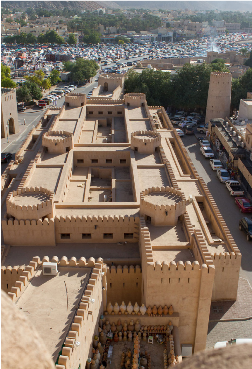
fig 2.20 | Nizwa Fort Market was designed to have a finish and look similar to historical structures by using Gypsum mud to finish the exterior of the market.
