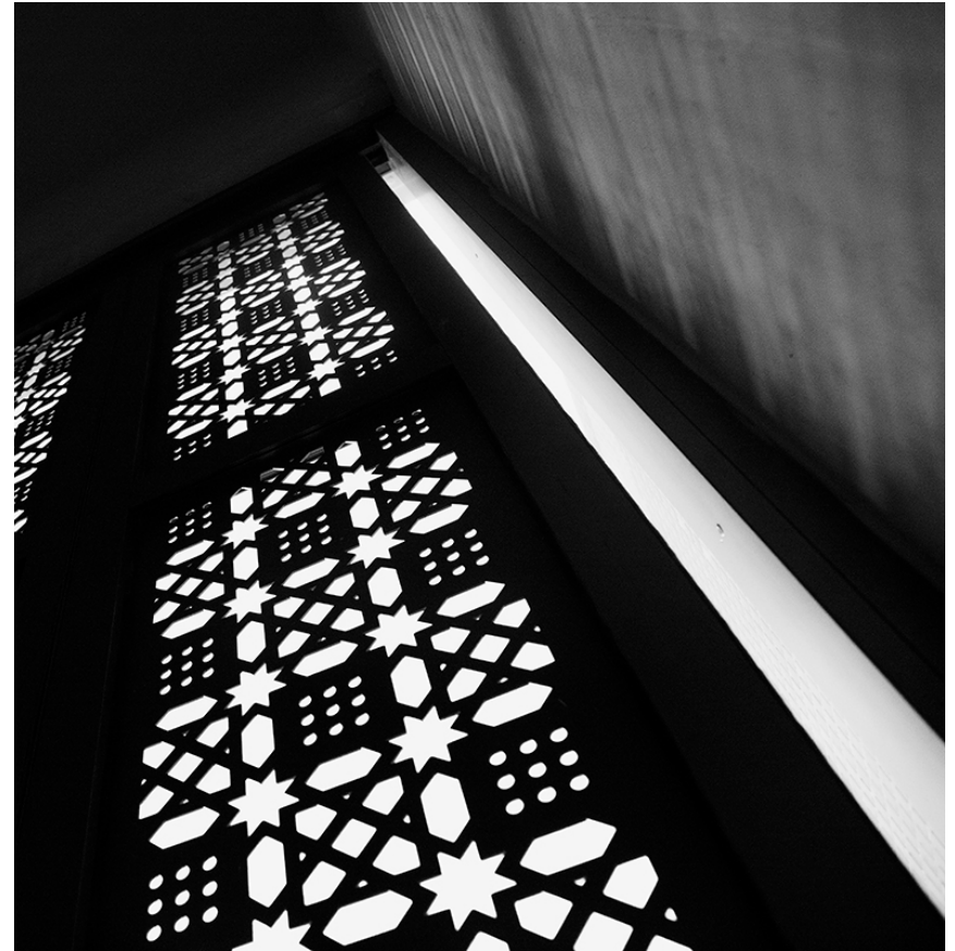
fig 2.21 | Decorative mashrabiya implemented in Mutrah fish market offer a cultural presence and define the identity of the space as well as function to reduce heat gain and direct sunlight.
