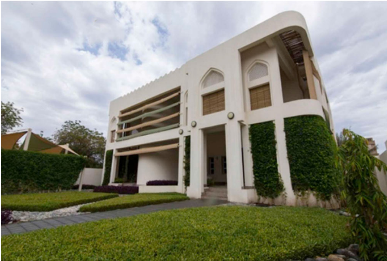
fig 2.17 | The Zero Energy Building Located in Sultan Qaboos University. Shading strategies are implemented on the exterior of the building to reduce heat gain and direct sunlight to the interior.
