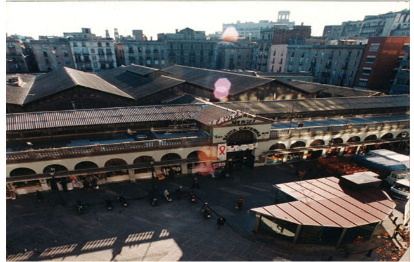
fig 2.11 | Santa Catrina Market old roof pre-renovation.
