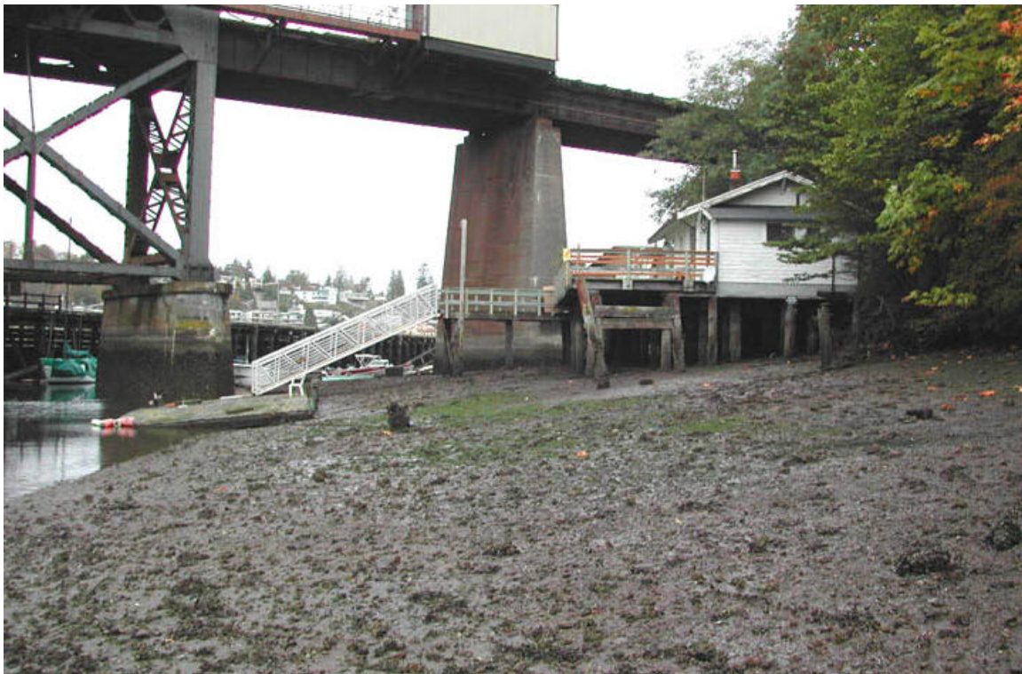
Figure 3. The Salmon Bay Natural Area study site at low tide, showing the overwater structure and floating dock.
