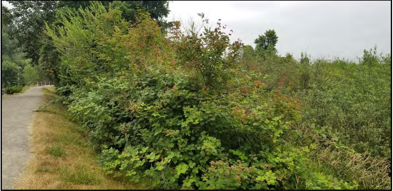
Photograph 9. East side levee looking south into the wetlands. (T. Allard, July 2, 2019)
