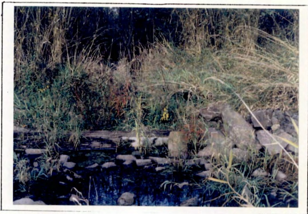
Photo #23 -- Log berm at south end of backwater wetland.
