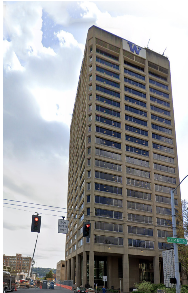
Figure 40. Before the Facade Renovation Image Source : Google Maps
