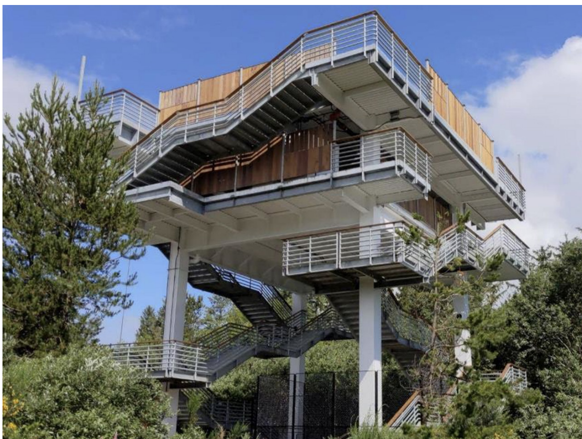
Figure 3. The Tsunami Vertical Evacuation Tower completed in 2022 that was funded and spearheaded by the SBIT in partnership with FEMA to support community resilience.
