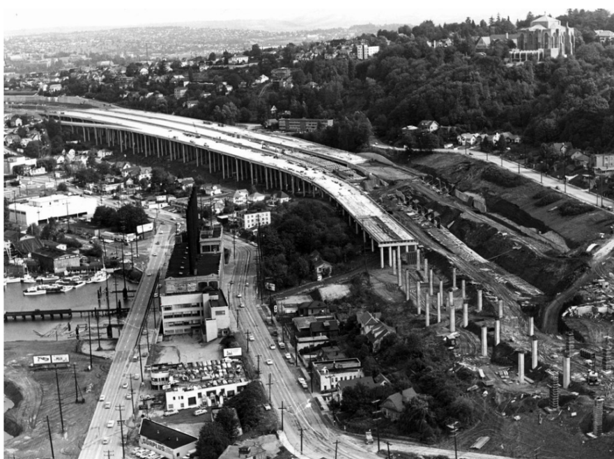
Figure 33 Construction of I-5 east of Lake Union
