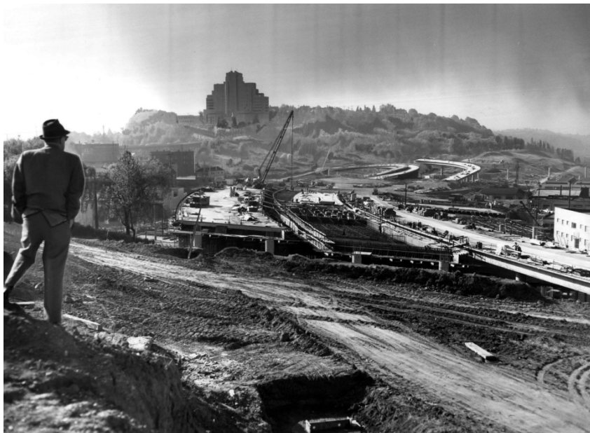
Figure 34 Construction of I-5 looking towards Beacon Hill
