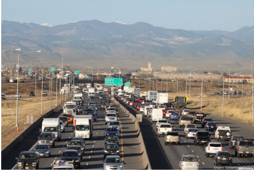
Figure 12 Denver's I-70 corridor
