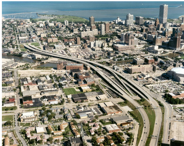
Figure 21 Park East Freeway, Milwaukee, WI before
