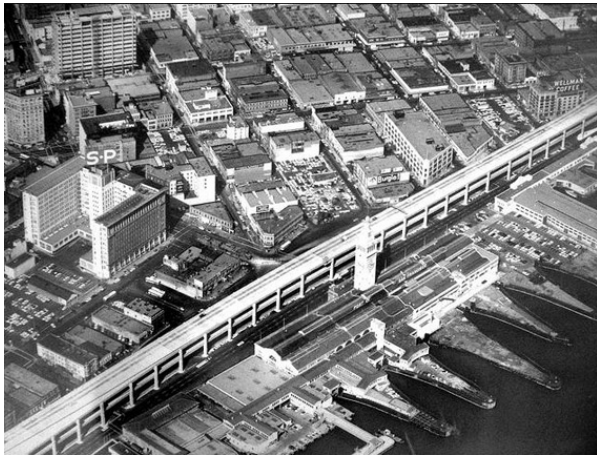
Figure 23 Embarcadero Freeway, San Francisco before
