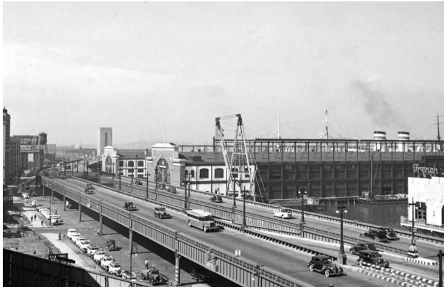
Figure 17 Westside Highway, NYC, NY Before
