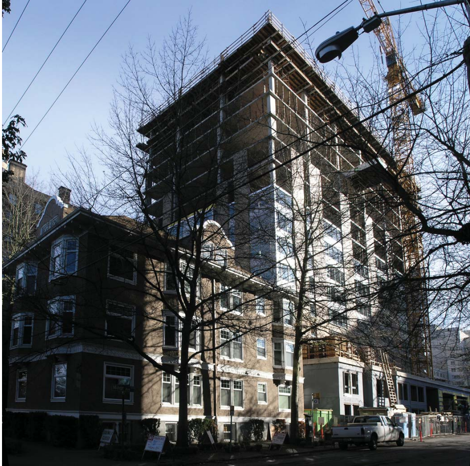
Figure 2.8 – 1200 Madison Street tower under construction (November 2011). Source: Sean Engle
