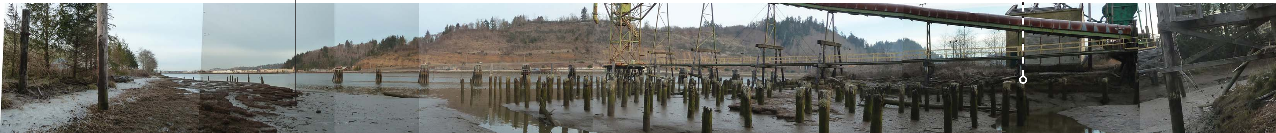
Fig. 4-32. Shannon Slough's soft and armored shores.
