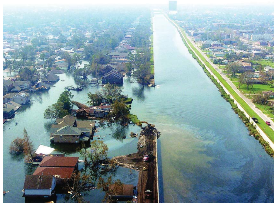
Fig. 3-44. 17th Street Canal breach, New Orleans, 2005. Resilience requires a move away from fracture-critical infrastructure. (image: nola.com)
