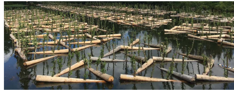
Fig. 3-23. Floating wetlands with an open structure promote dappled light penetration and salmon refuge at Brightwater Treatment Plant, Woodinville, Washington. (image: MacDonald 2016)
