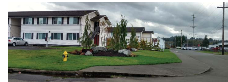
Figs. 3-19, 3-20. South Aberdeen apartments elevated on a berm (top) allow flooding around the perimeter. Not much adaptive development like this exists as new local real estate investment is minimal. BIG’s “Dry Line” creates protective and recreational transition zones between urbanization and water (image: Lafarge Holcim Foundation)
