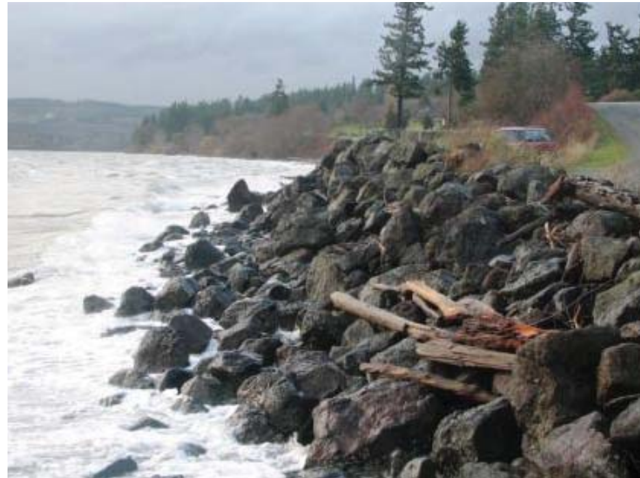
Fig. 3-11. Typical rip rap revetment. (image: ecy.wa.gov)
