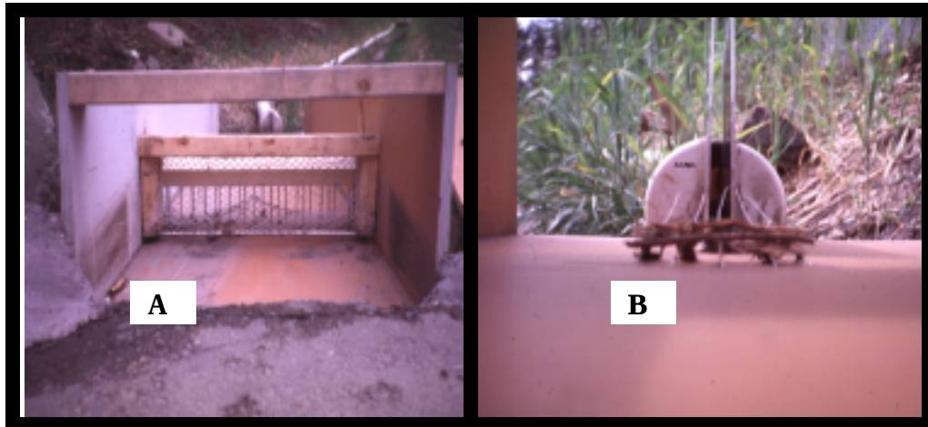
Figure 3.8 (A) Inclined netting and inverted rake at splitter inlet (B) Aluminum wire rack immediately upstream of diversion channel
