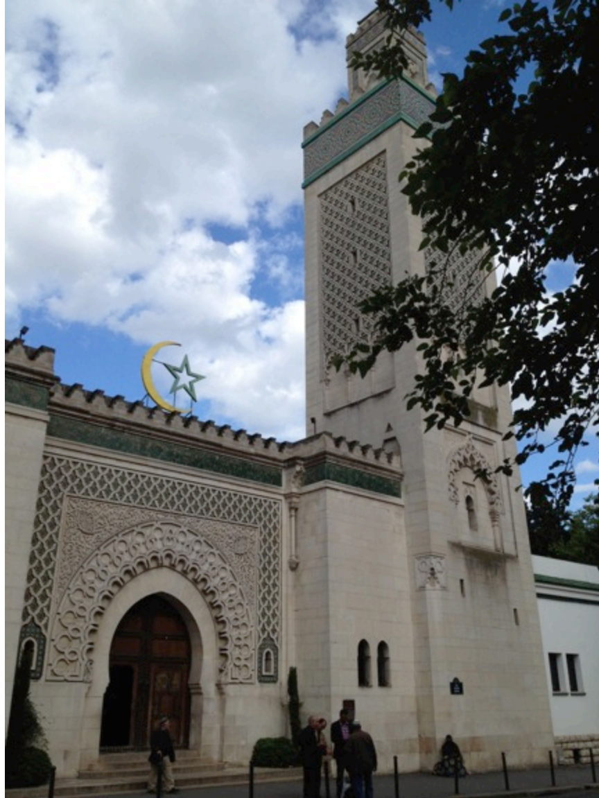
Figure 8.6 Entry, Great Mosque of Paris
