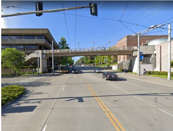
Figure A.1 Existing pedestrian bridge
