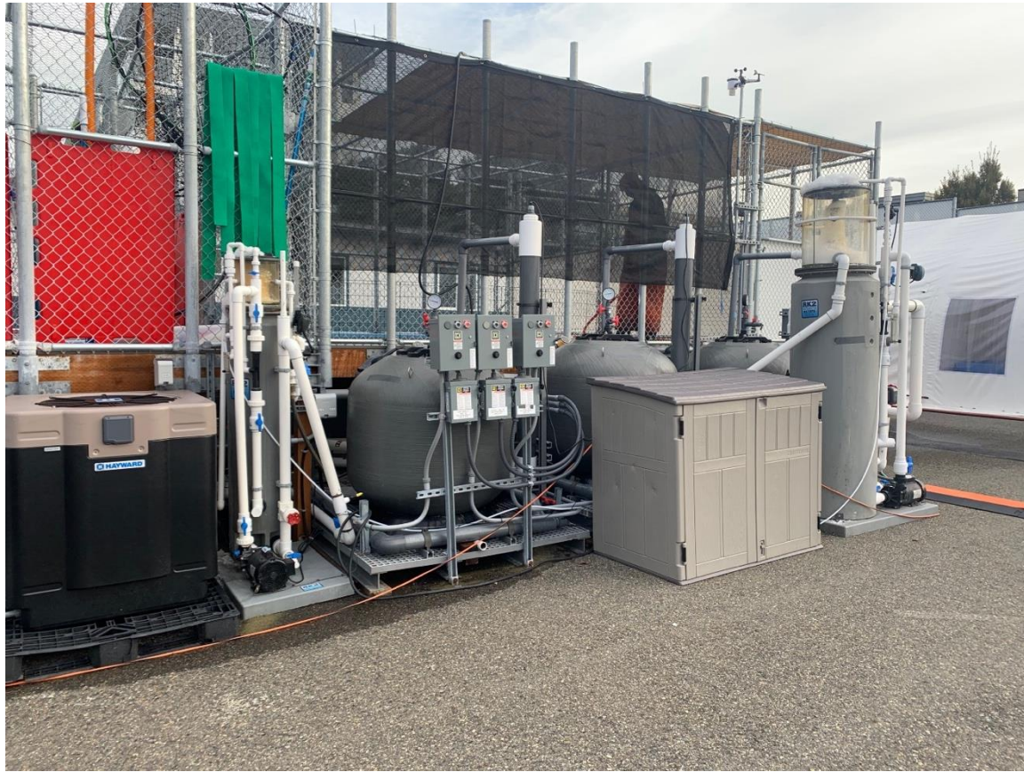
Image 2. Water treatment system components. The two towers are the ozone contact basins. The weather station was mounted on top right the fence of the pool deck and remained in the same location for the entirety of the study. The zone 1 ozone measurements were collected adjacent to the left (smaller) tower.
