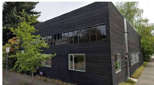
Existing Commercial (SE corner of 56th St. and 1st Ave)
