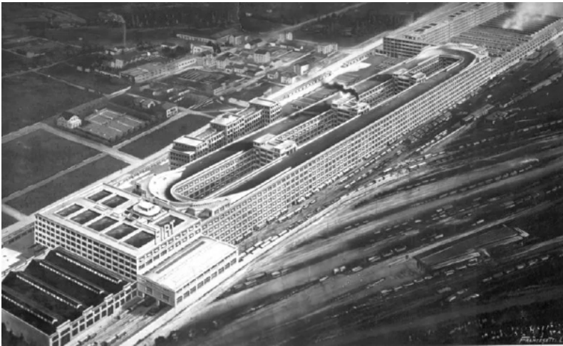
Figure 2-7. Giacomo Matte-Trucco, Fiat Factory, 1927. The Fiat Factory is a car assembly plant. The entire building is scaled to the size of a car, and they can be driven to any location in the 3.5 million square foot factory. The assembly line moves up in a continuous spiral, ending at a 1.5 mile long rooftop testing track.
