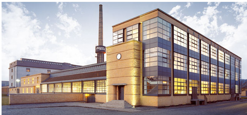
Figure 2-6. Walter Gropius, Faguswerk, Alfeld, Germany, 1911. This building defined the modern “factory aesthetic.” Gropius pushed the capabilities of new building materials, a feeling of weightlessness was achieved through expansive use of glass, and the corner showcases the cantilevered stair.
