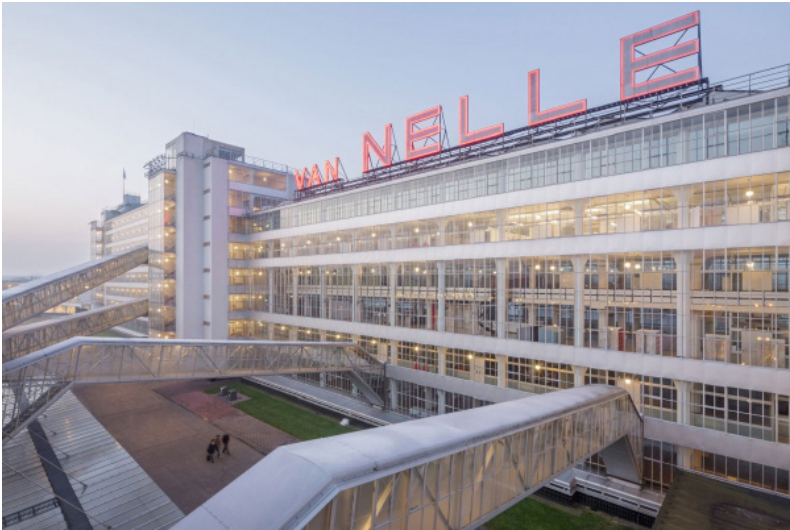
Figure 2-19. View of the conveyor belts between buildings.
