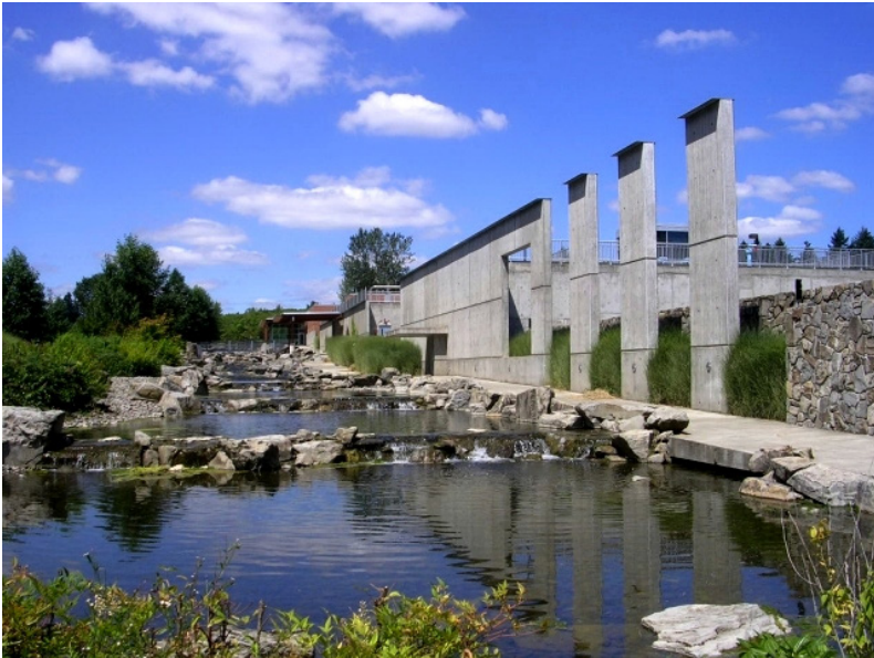
Figure 2-24. Ponds on the public side of the wall.
