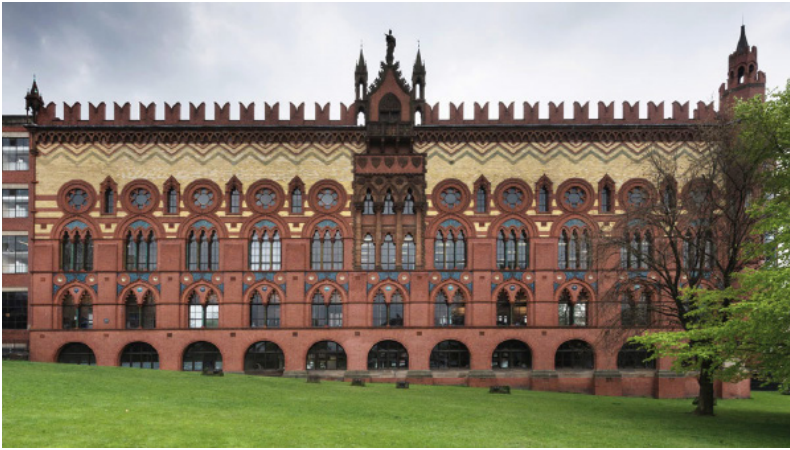
Figure 2-3. The Glasgow Carpet Factory, James Templeton, 1889. The lavish ornament was meant to evoke the similarly decorative carpets that the factory produced, and thus the factory building itself served as an advertisement for its product. Factories of this period often used historic styles of decoration on the new typology. Templeton based the facade design on Ruskin's drawings in The Stones of Venice .
