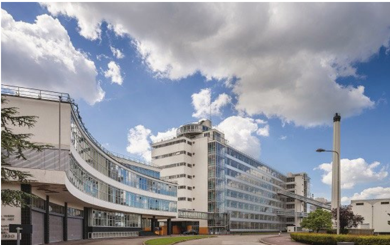
Figure 2-8. Brinkman & Van der Vlugt, Van Nelle Factory, Netherlands, 1931. This factory celebrated new technology, using unbroken glass facades and hovering conveyor belts to move goods and people between buildings. It also included sports facilities, a garden, and a library for its employees.
