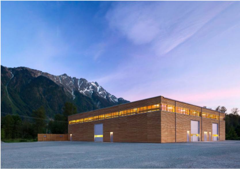
Figure 2-17. Exterior of the Passivhaus Factory.
