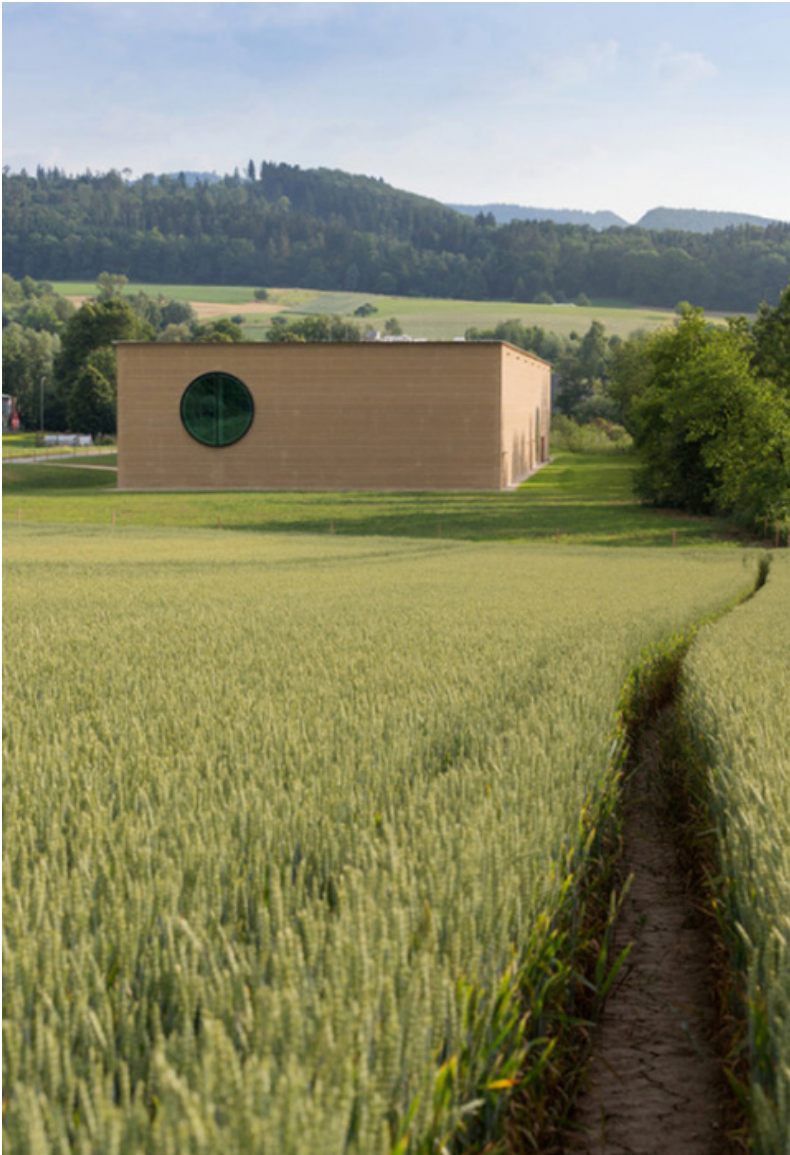
Figure 2-21. Rammed earth facade and viewing portal into the Ricola Herb Factory.
