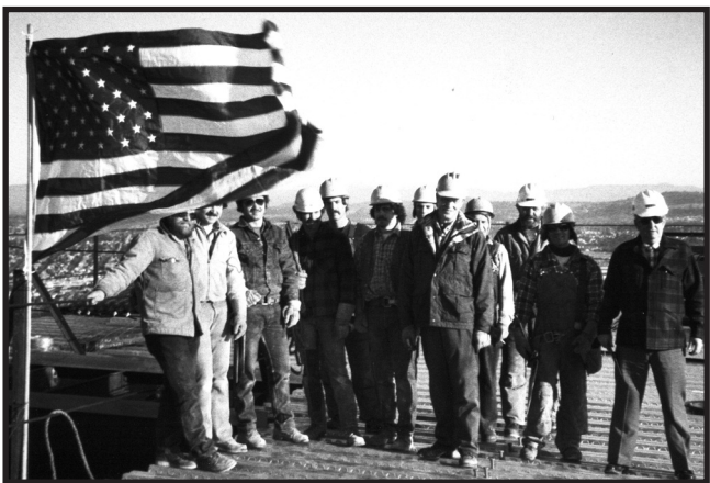
Members of Iron Workers Local 29 pose atop the new Veterans Administration Hospital on "Pill Hill" in Southwest Portland in February 1984.
