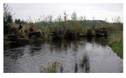
In summer 2001, restoration construction diverted North Creek into a new channel and reestablished 58 acres of early successional floodplain forest. The old channelized section of creek was filled in and transformed into a tributary wetland complex. The new channel was designed to allow the river to re-meander across the floodplain (within project constraints) and overflow its banks approximately once every year.
