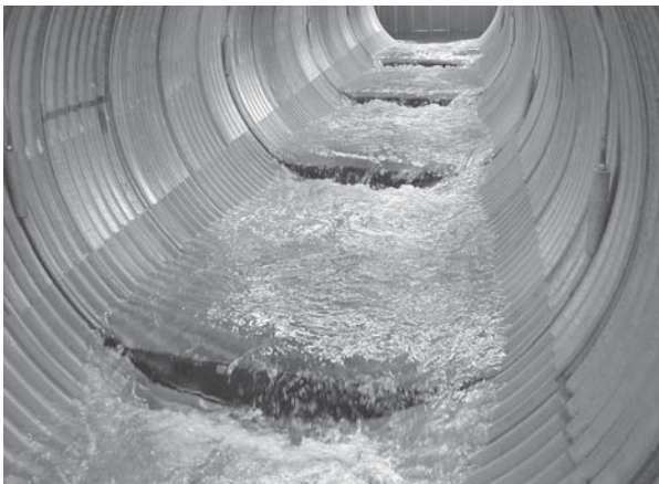
Above: Baffled culvert test bed near Tenino, Washington.
