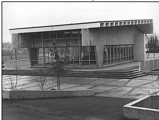
Figure 15 • West and east façades, 1963
