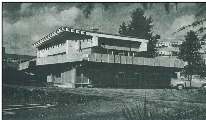
Figure 14 • View of south and east façades, 1963
