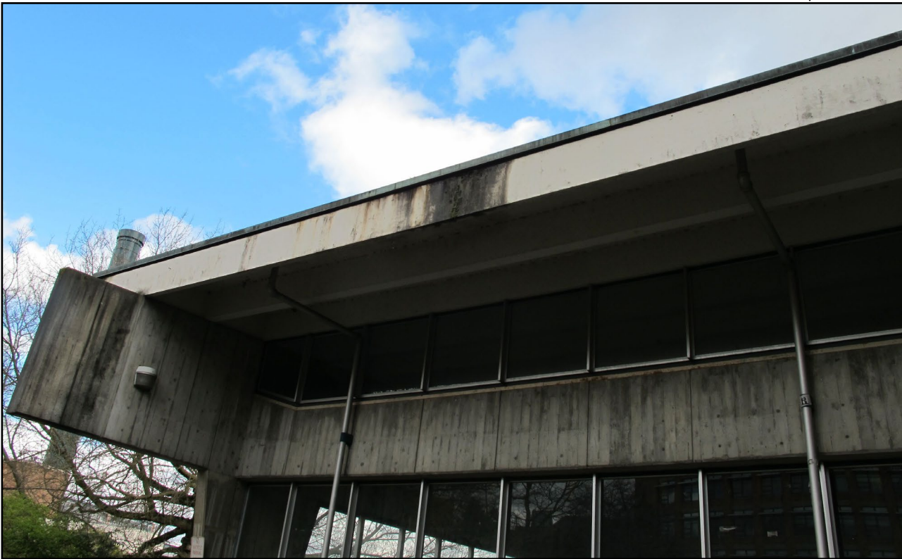
Figure 4 • More Hall Annex, detail of western façade overhang
