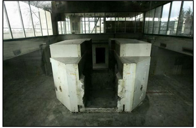
Figure 11 • Reactor room, viewing east from exterior
