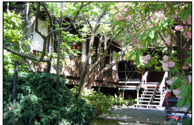
Figure 51 • Zema Office Building and Japanese Antique Gallery, Eastlake and Boston, Seattle, Zema, 1968
