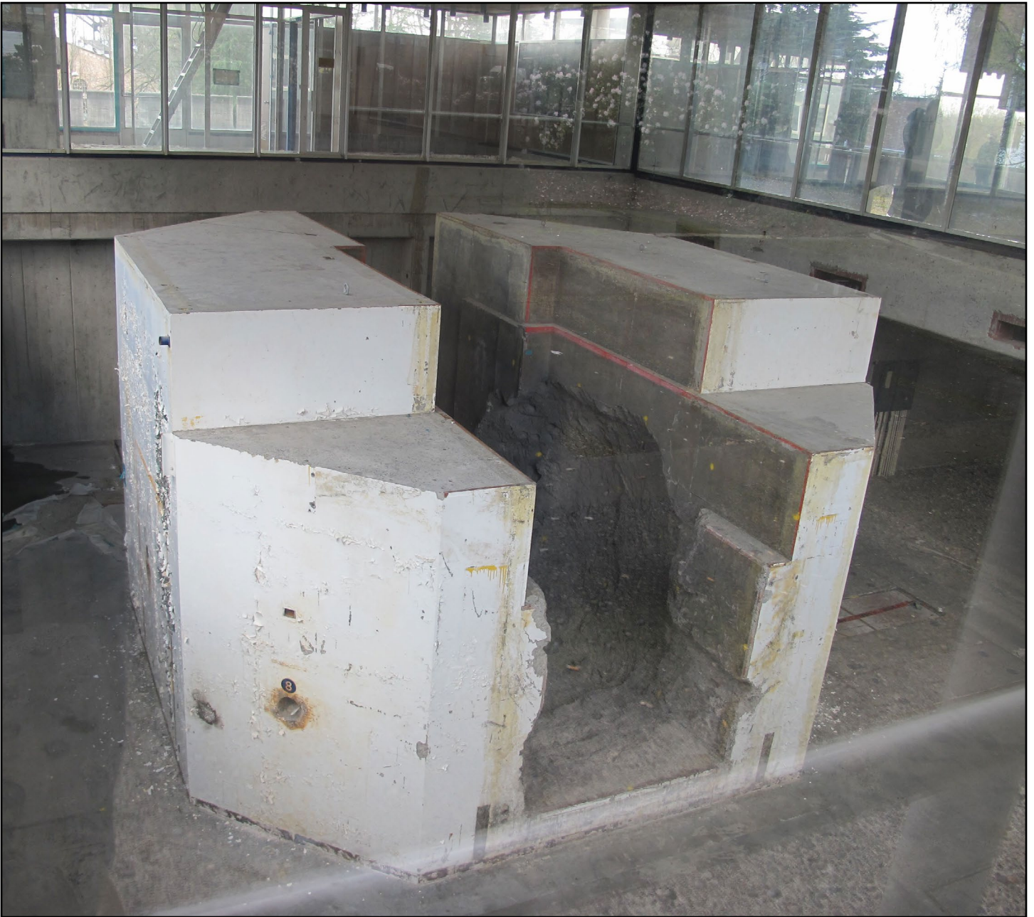
Figure 6 • More Hall Annex, viewing southeast into decommissioned reactor core
