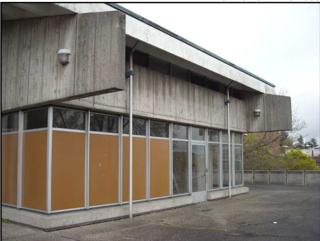
Figure 8 • East and partial south façades
