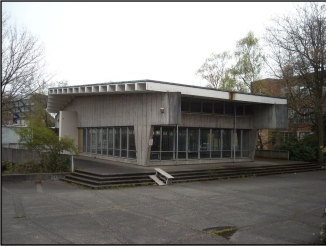
Figure 4 • North and west façades
