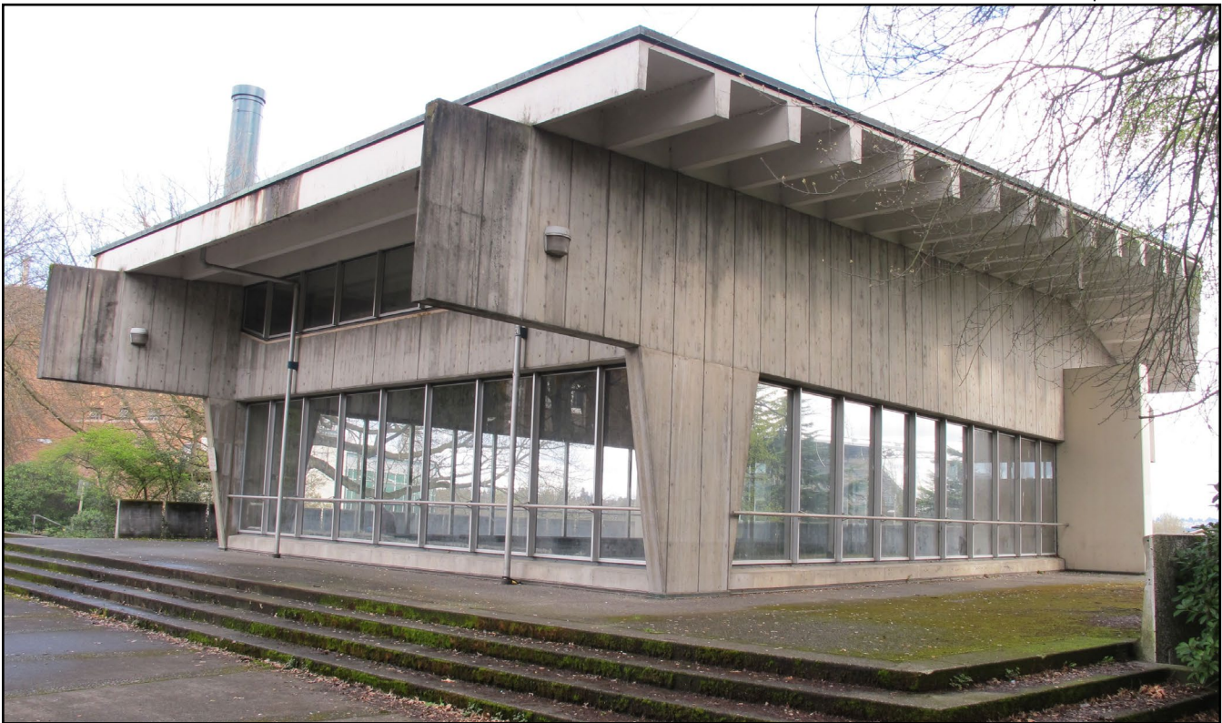
Figure 2 • More Hall Annex, northern and southern façades
