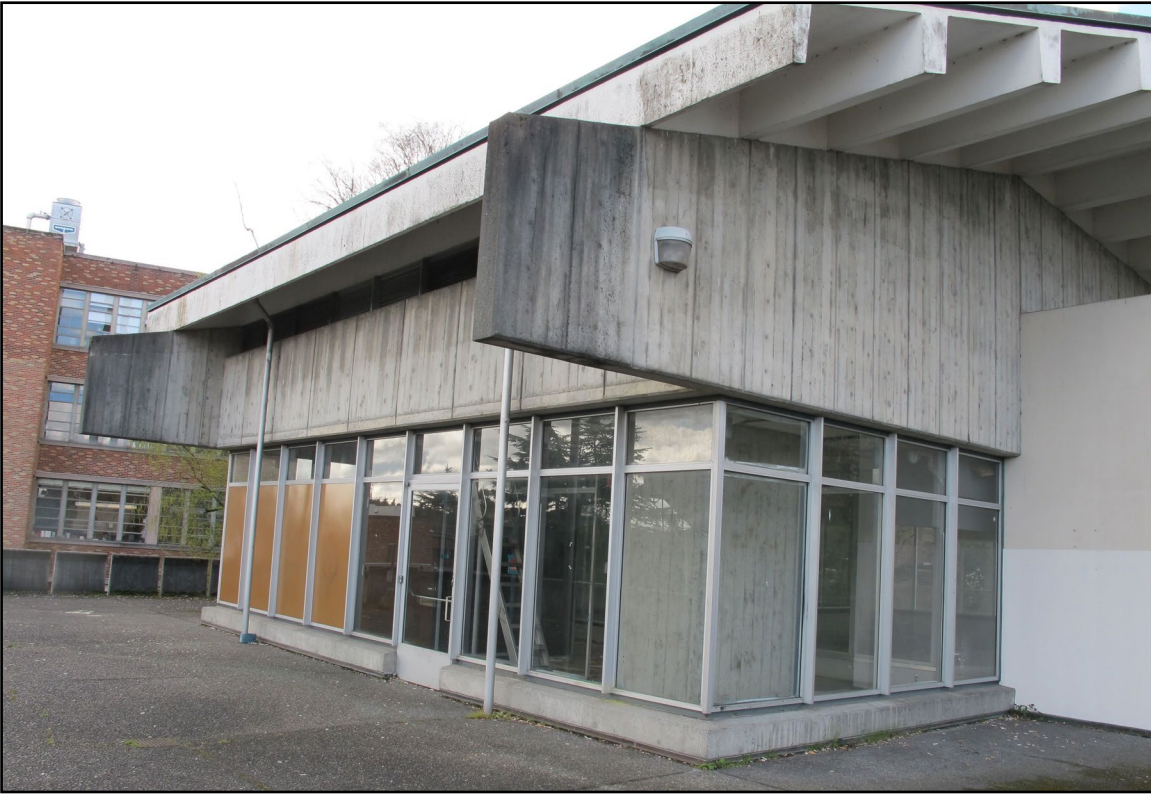
Figure 3 • More Hall Annex, eastern façade
