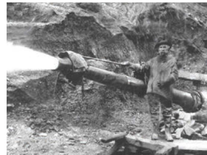
Figure 3.2 Hydraulic mining “Giant” in California (Salmon River Restoration Council Archive / Dobson Collection)
