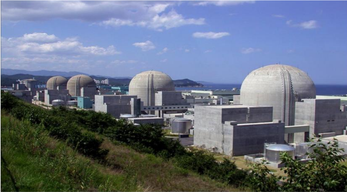
Figure 7.8. Ulchin Nuclear Power Plant, South Korea (OPR-1000s)
