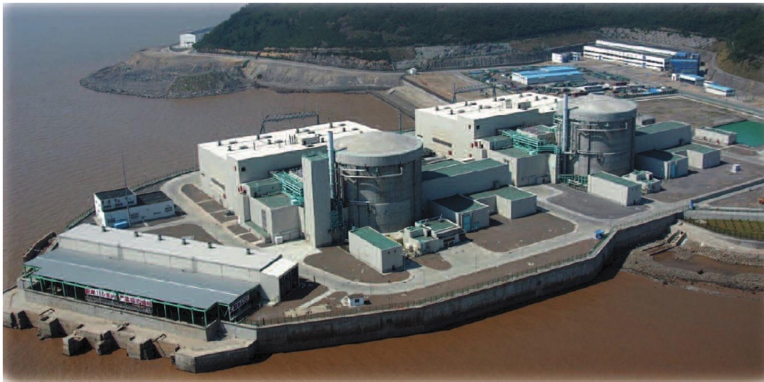
Figure 7.6. Chinese Qinshan Power Plant Phase III, Units 1 and 2 (CANDU 6 reactor)
