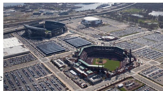
Figure 6. Philadelphia Stadium Area
