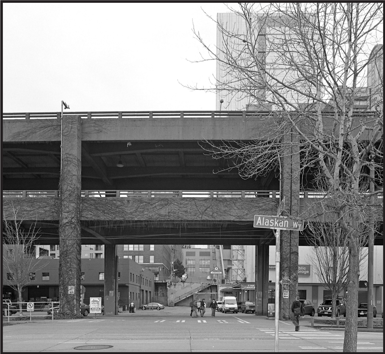
Figure 14: Pedestrian Visual Barriers to the Waterfront Source: Author
