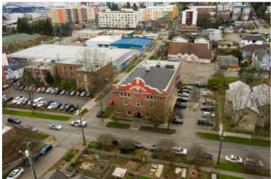
Figure 5 Aerial Photo of Washington Hall
