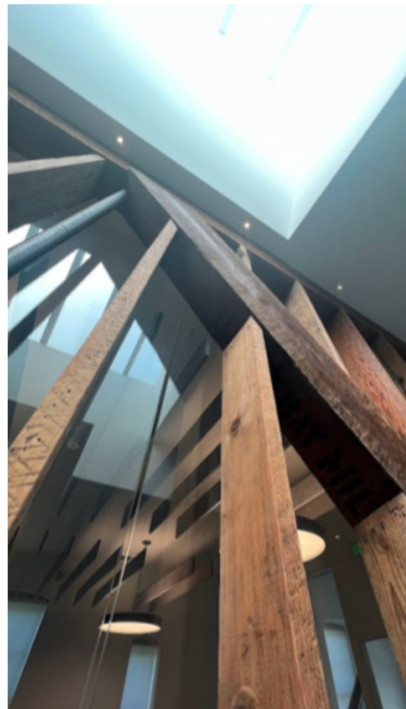
Figure 18 Original timber beams separate the upstairs elevator lobby with overhead skylight from the office space with acoustical panels in ceiling Source: Michelle Bacca
