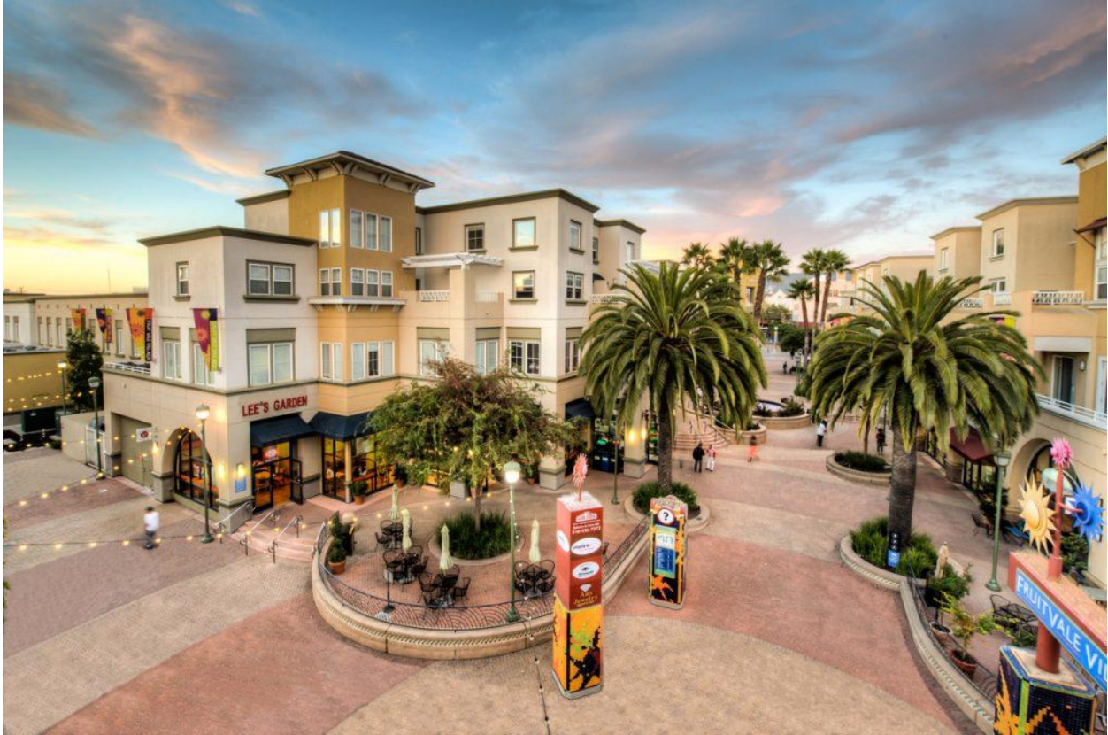
Figure 13: Fruitvale Village Plaza, https://pgadesign.com/projects/fruitvale-transit-village/
