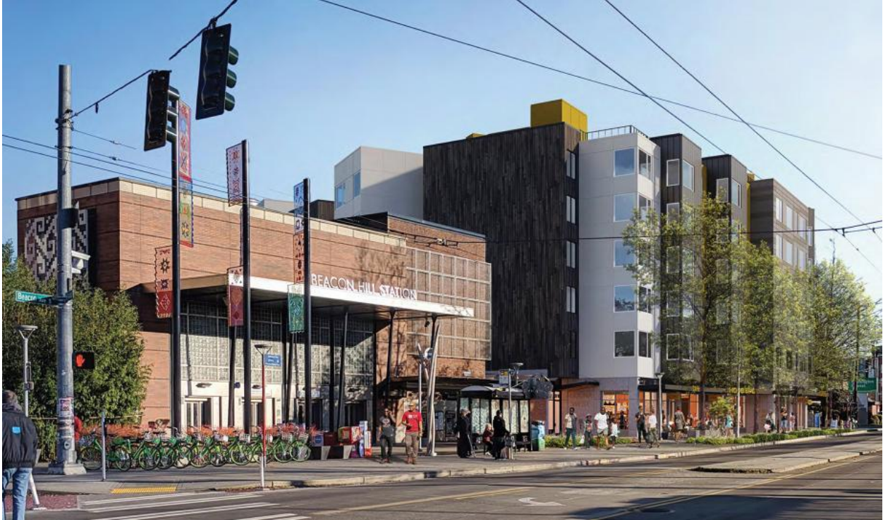
Figure 19: Beacon Hill Light Rail Station with the Colina Apartments just behind, https://www.soundtransit.org/system-expansion/creating-vibrant-stations/transit-oriented-development/beacon-hill
