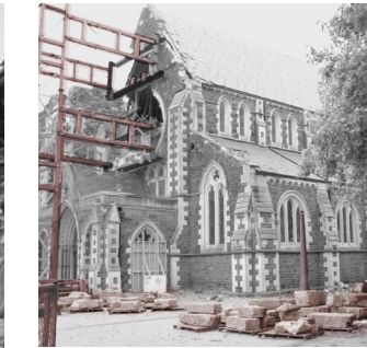
Old Stones & Construction Materials Will be replaced or reused.
