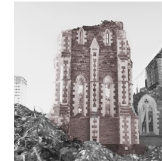
Bell Tower Will be rebuilt.
