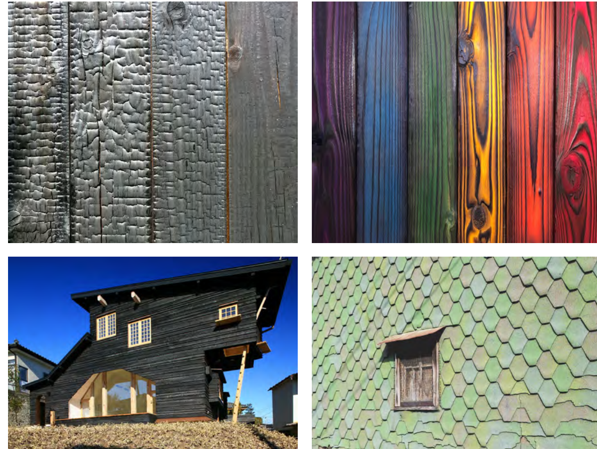
Fig. 45, 46, 47 & 48 - A variety of yakisugi treatments of wood, to include rough char to sanded and color treatments. Now imagine the beauty of scales and reuse in combining the bottom images. Rigged up with a fresnel lens or utilizing fuels produced through the gasification or biodigestion processes, the charring of the wood itself can be considered carbon neutral.. Photos: (top left, bottom left) "yakisugi," 2020; (top right) Vespa, 2018; (bottom right) Haanala 76, 2020.
