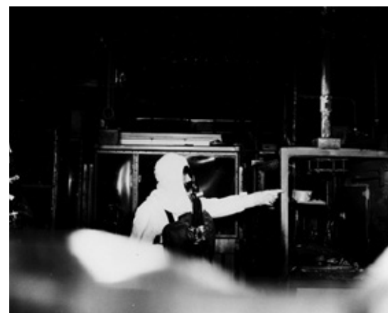
Figure 42 | Damage from the 1957 Fire
