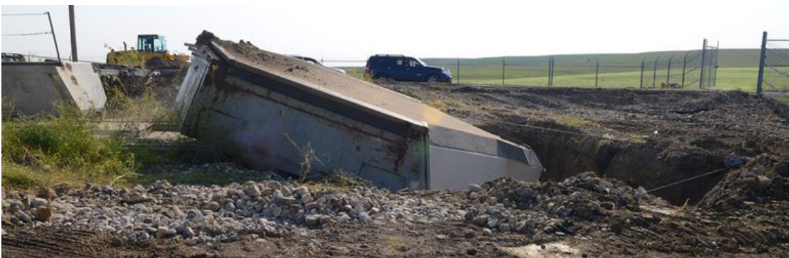
Figure 6 | The demolition of a Minute Man II Missile Silo
