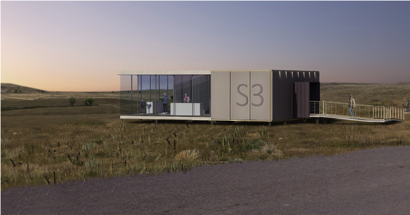
Figure 74| View of Surface Monitoring Station 3 Exiting the Site
