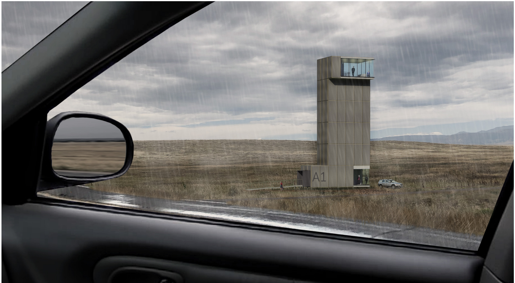
Figure 66 | View Approaching the Air Monitoring Station
