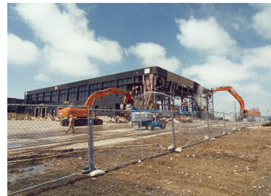
Figure 5 | Demolition of Rocky Flats
