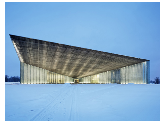
Figure 22 | View of Exterior & Entry Canopy
