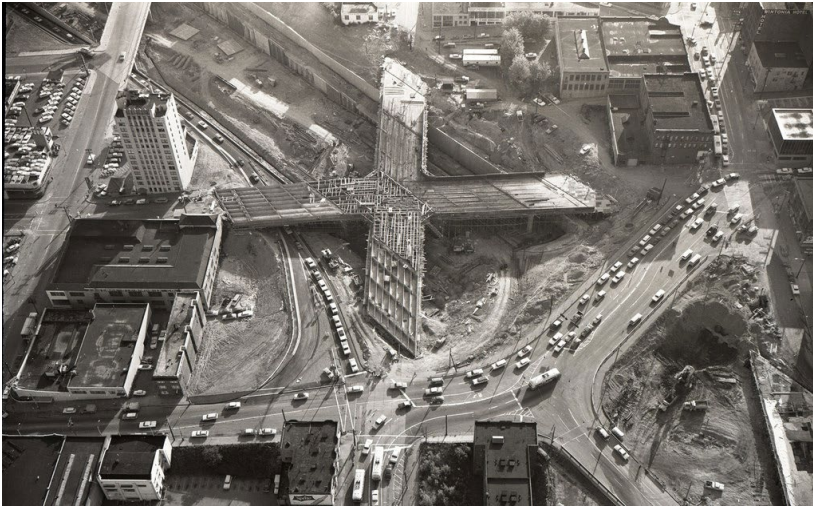
Figure 10. Construction of the Freeway
