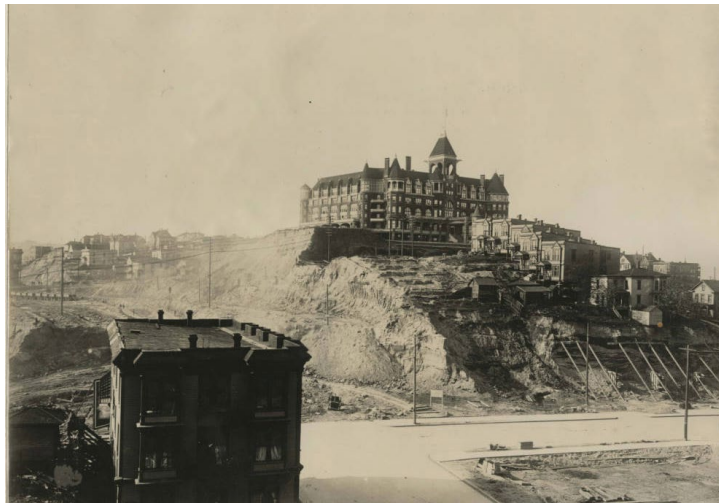
Figure 8. View of regrade work north from 2nd Ave. and Pine, ca. 1906
