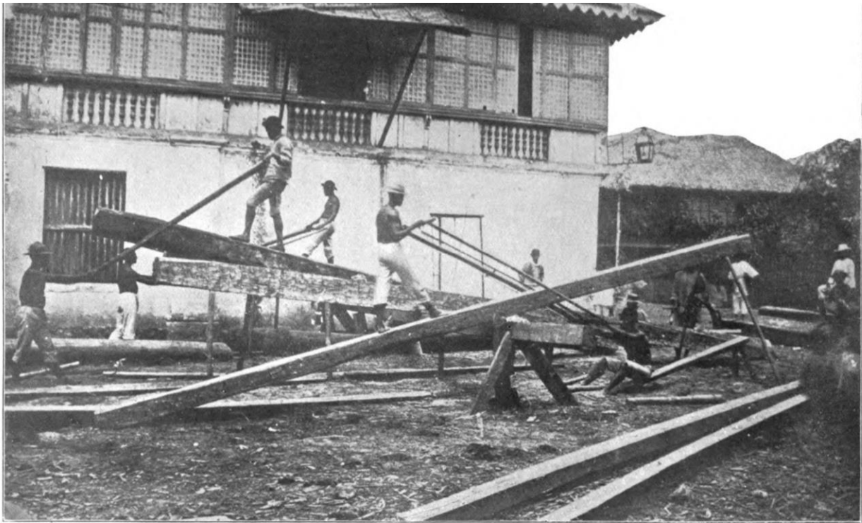
NO. 10. RIPPING OUT BOARDS IN THE CITY OF MANILA.
