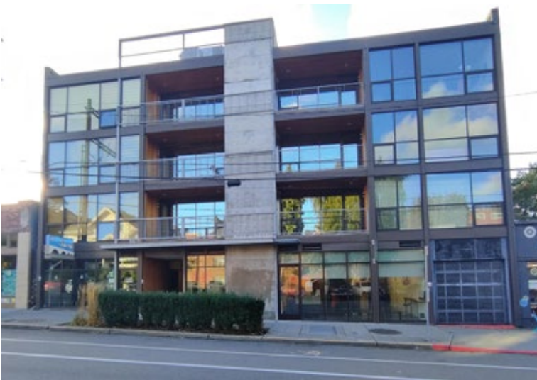
Figure 47: Park Modern: 5612 University Wy NE. (Build LLC). Symmetry, carved porches.
