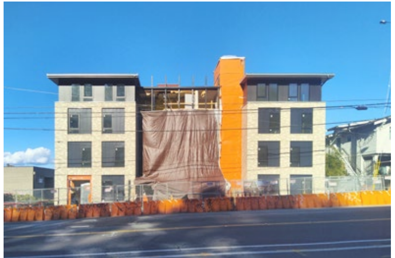
Figure 8: image of 2514 Dexter Ave N under construction in spring of 2023.
