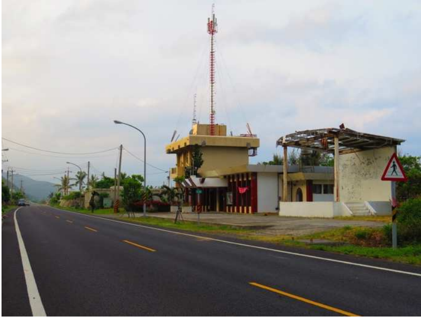
Figure 11 “A crumbling community center” of Nantian Village by the new Highway 26,
