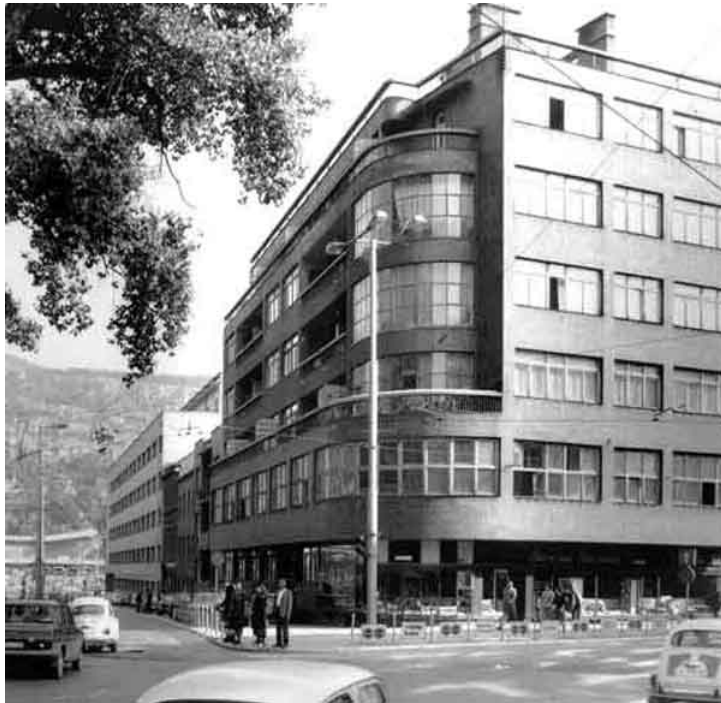
Figure 17: Muhamed and Reuf Kadic, Building of the Pension Fund, Sarajevo, 1940, Courtesy of www.a4a.info
