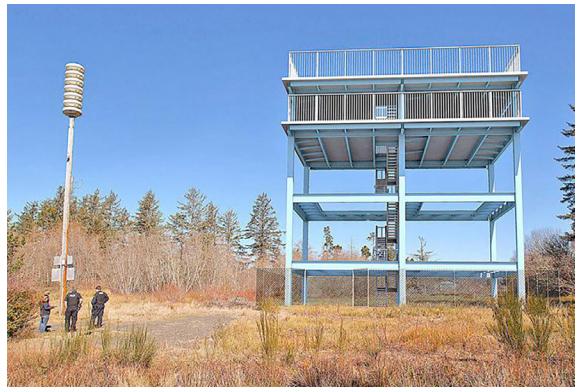
Figure 21. Rendering of a new tsunami evacuation tower for the Shoalwater Bay Tribe near Tokeland, WA. Image by Visual Engineering Resource Group via Chinook Observer ( Design Work Underway for Shoalwater Tsunami Evacuation Tower 2019).
