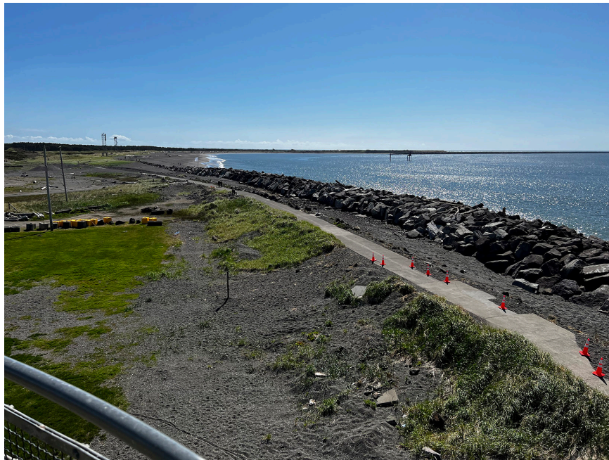
Figure 49. Rock wall beach armaments along the northern coast of Westport. Photo by Brook Goodwin (2022).
