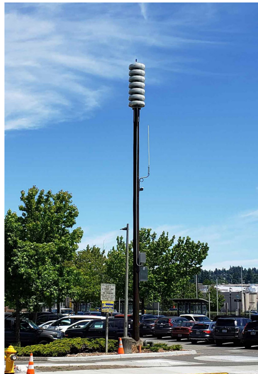
Figure 20. A tsunami warning siren in Edmonds, WA. Photo by Everett Post ( Outdoor Tsunami Warning Sirens Coming to the North Sound 2021).
