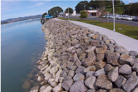
Figure 18. A beach armament installation made of large rock rip-rap in Tauranga, New Zealand. Photo by Cirtex Industries ( Tauranga Sea Wall Rock Revetment – TerraTex K Geotextile 2018).
