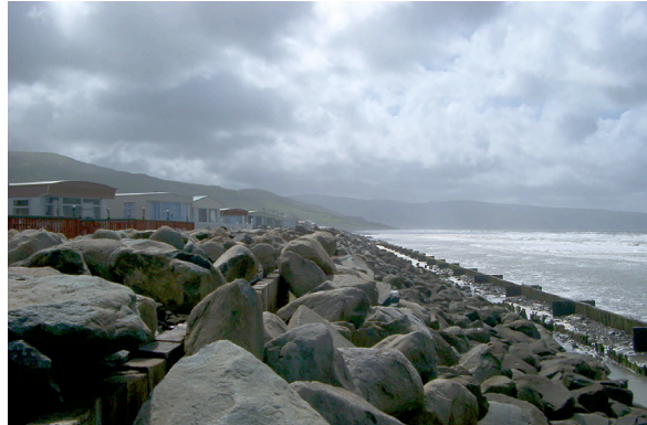
Figure 19. Beach armament made of heaps of large boulders in the UK. Photo distributed under CC BY 2.5 license via PhotoEverywhere.co.uk ( Sea Wall Coastal Defense 2008).
