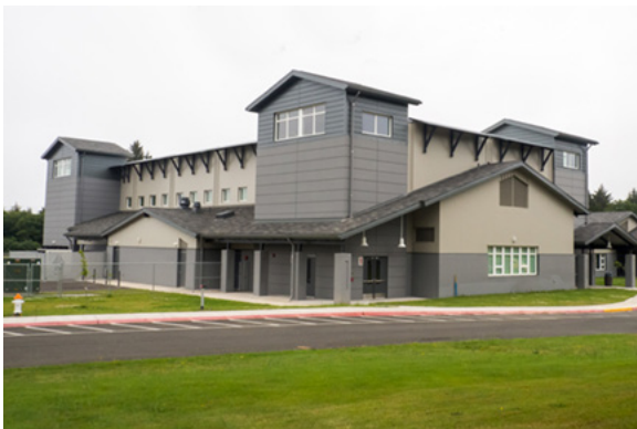
Figure 22. The first vertical tsunami evacuation structure was built as part of a new elementary school in the Ocosta School District in Westport, WA. Photo via WA DNR ( Tsunamis / Preparation and Evacuation / Vertical Evacuation n.d.-a).
