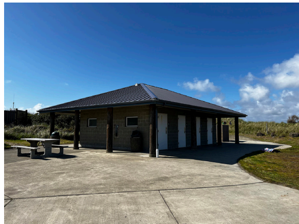
Figure 54. Restroom building at the northwestern corner of Westport Light State Park. Photo by Brook Goodwin (2022).
