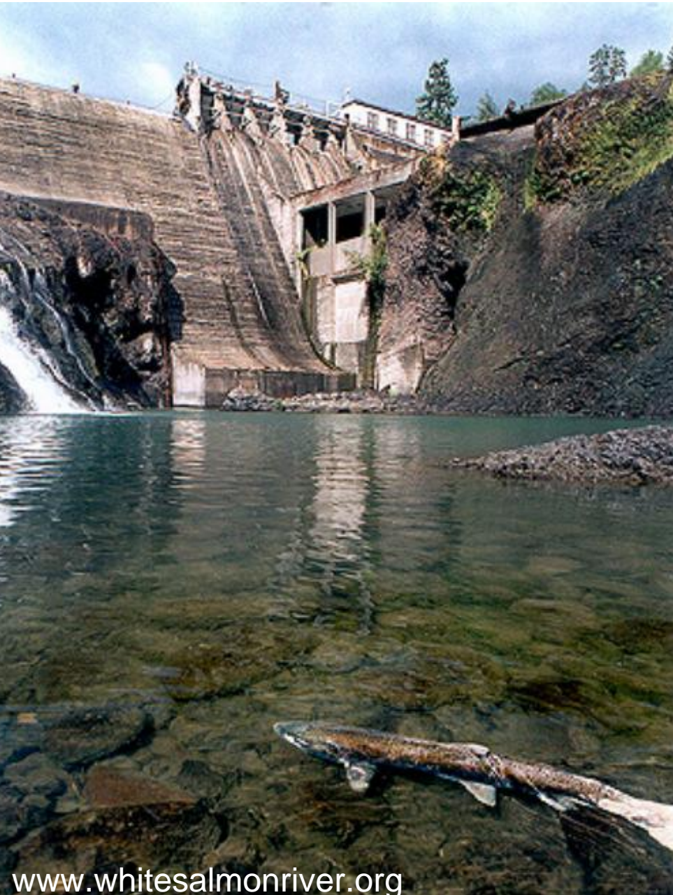
Condit Dam, White Salmon River, WA
