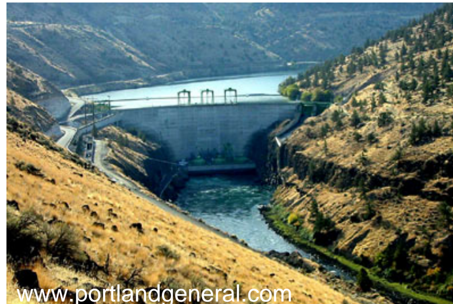
Pelton Dam, Deschutes River, OR
