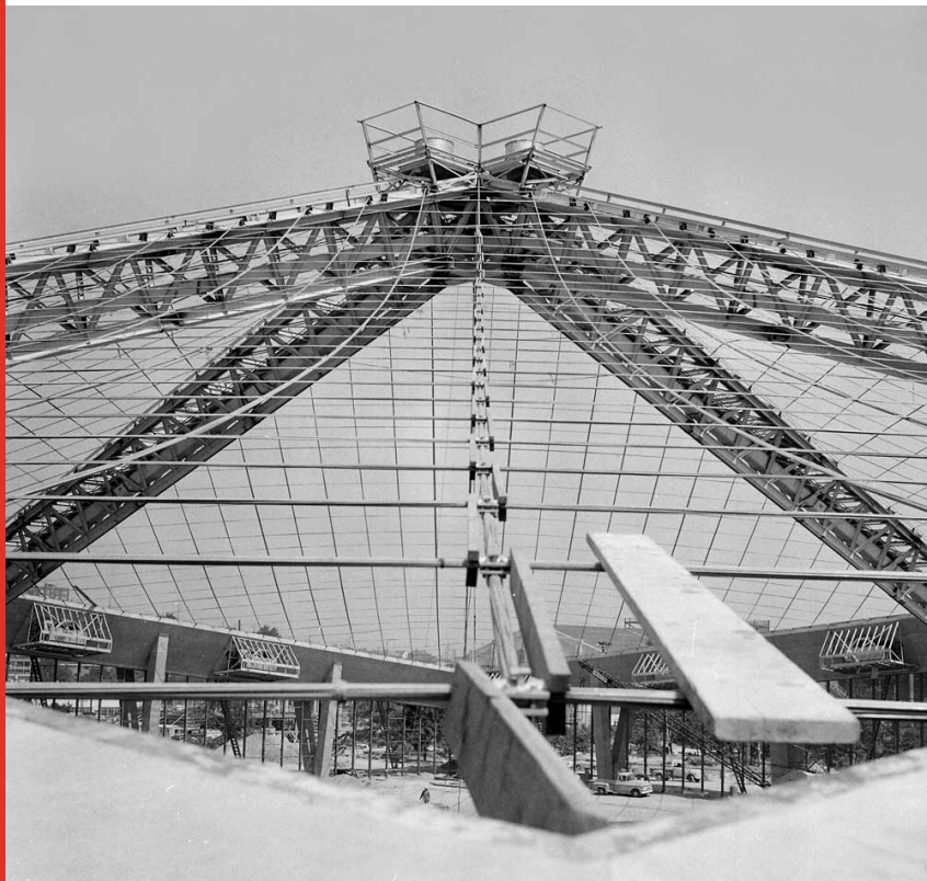
Victor Lygdman's construction stage photograph of the Coliseum's roof.
