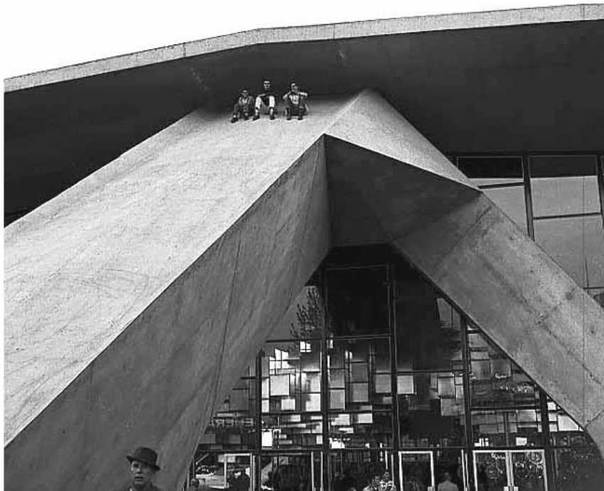
The three-legged gigantic concrete abutments from the exterior.
