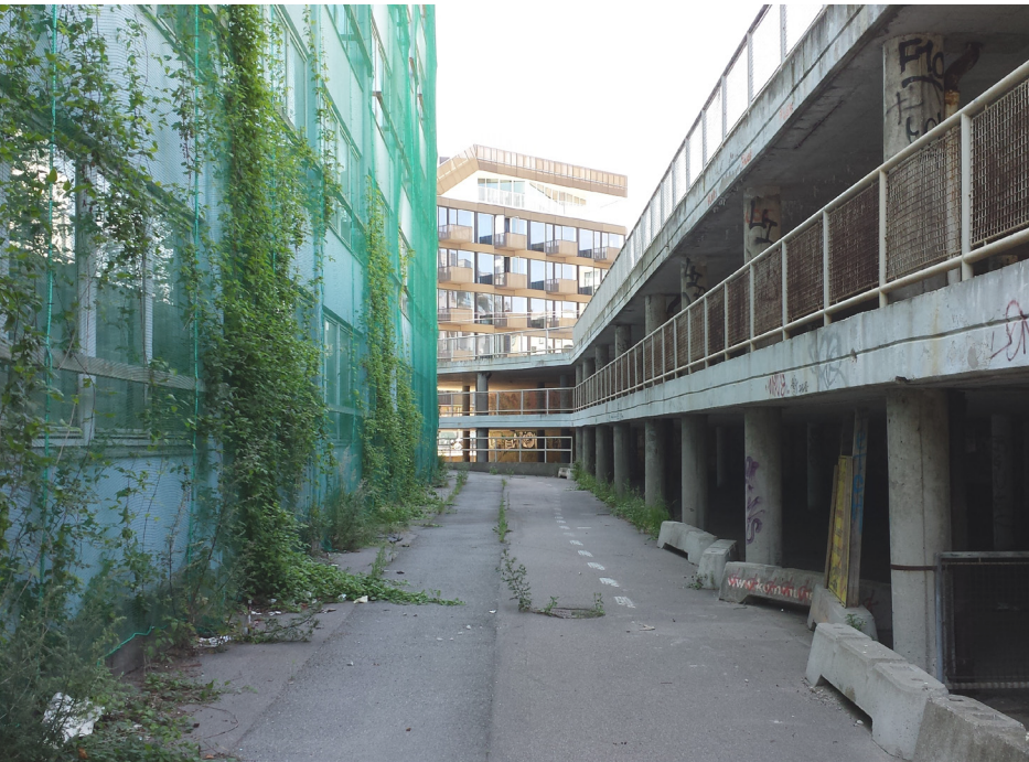
Figure 95. L. Between the parking garage and school, looking West
