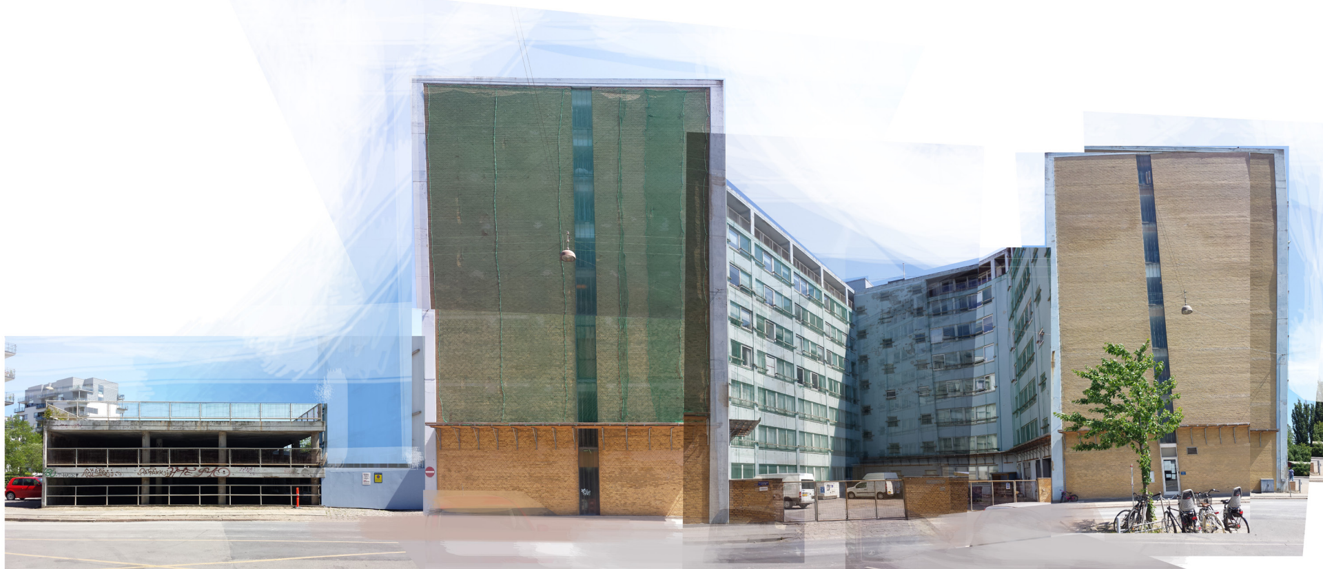
Figure 90. G. Abandoned School and parking garage, looking East
