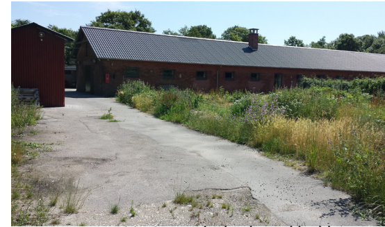
Figure 100. Q. Residual industrial building
