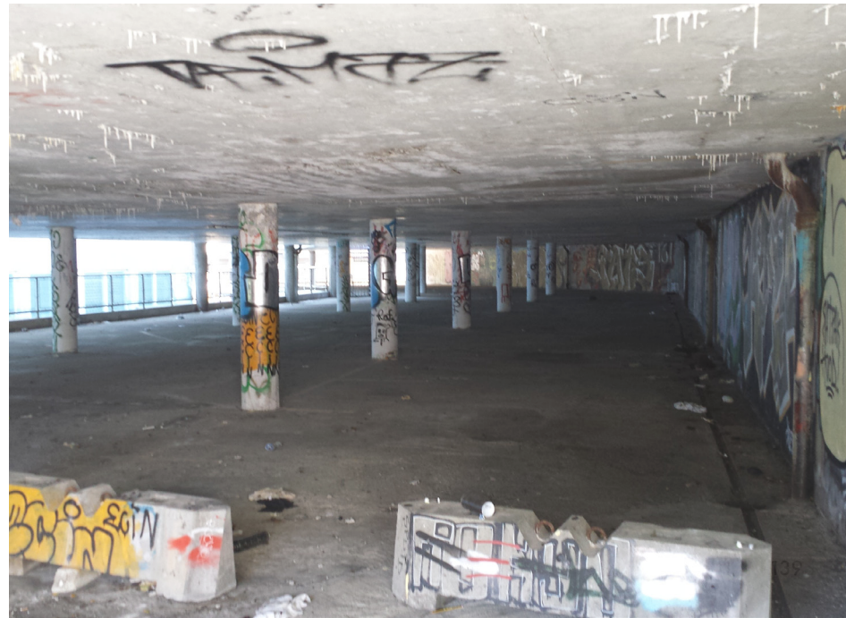
Figure 97. N. Concrete columns and floor plates
