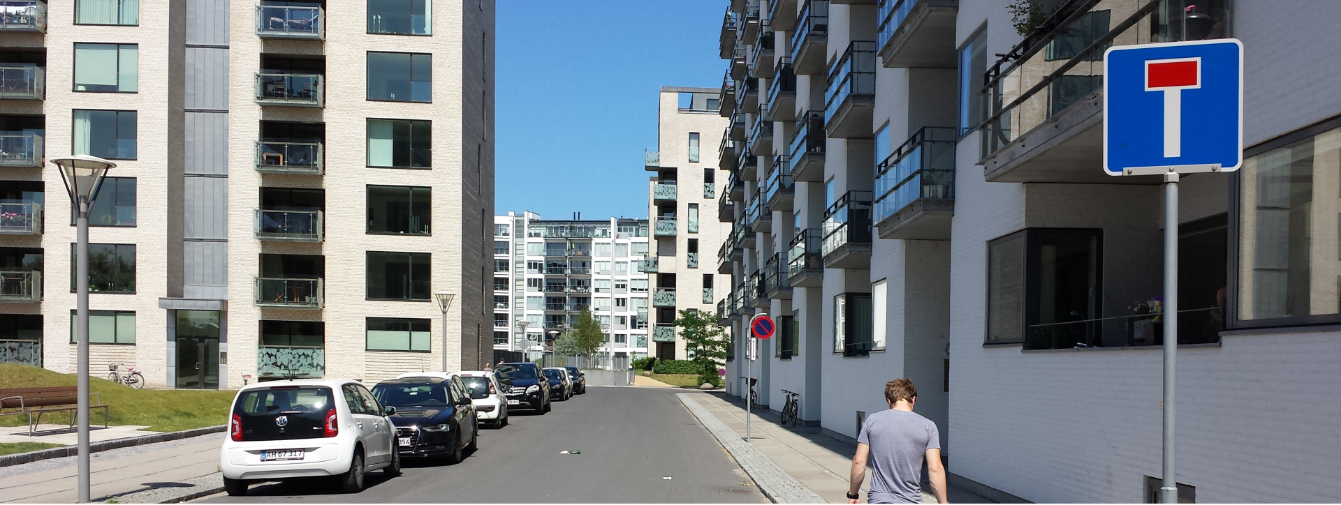
Figure 86. C. Looking North, access road to parking and courtyard
