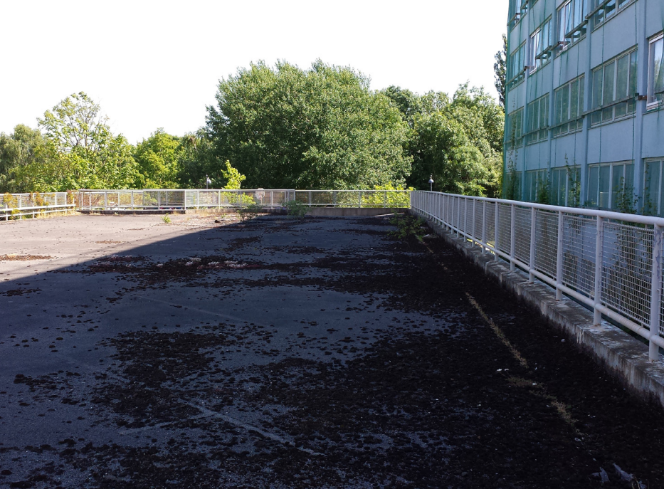
Figure 94. K. On top of the abandoned parking garage
