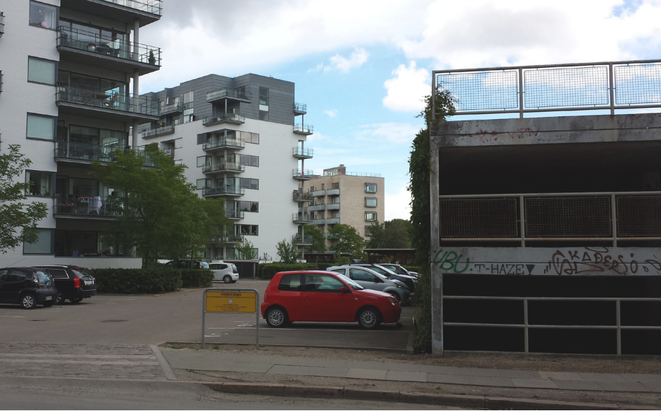
Figure 88. E. Streetscape and abandoned parking garage
