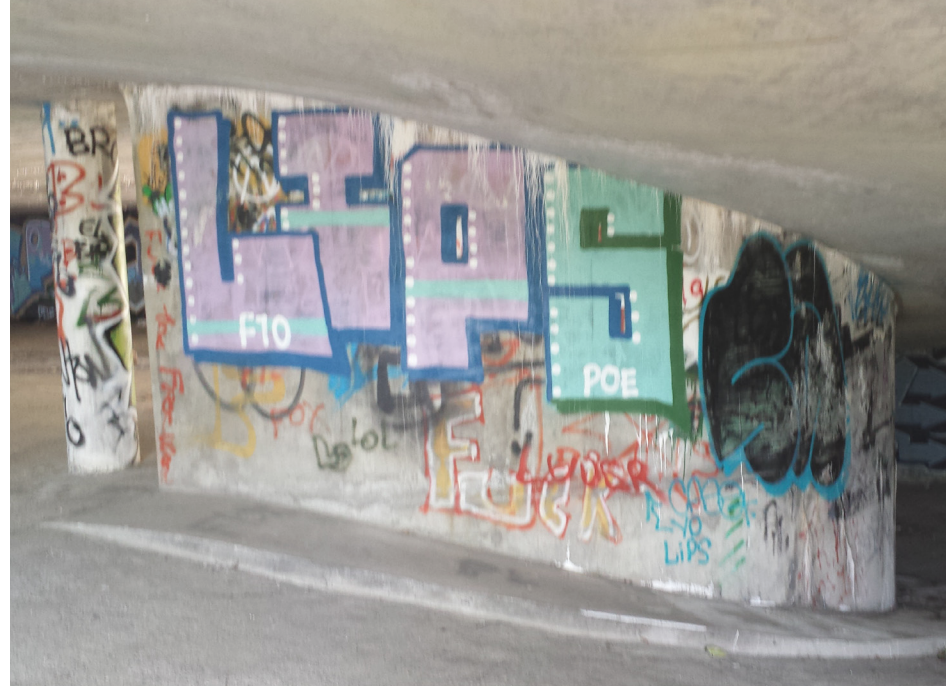
Figure 96. M. Parking garage interior round-about
