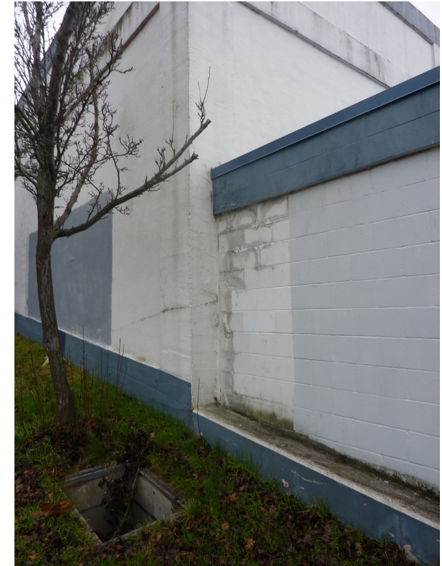
Figure 47: Containment wall detail along Woodlawn Avenue N., 2013.
