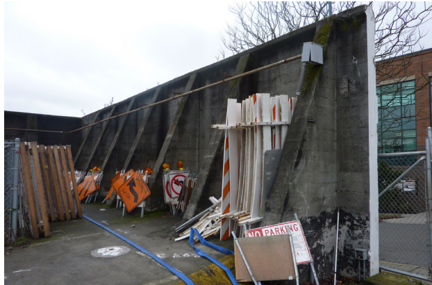
Figure 44: The buttresses of the containment wall facing the interior courtyard. 2014.
