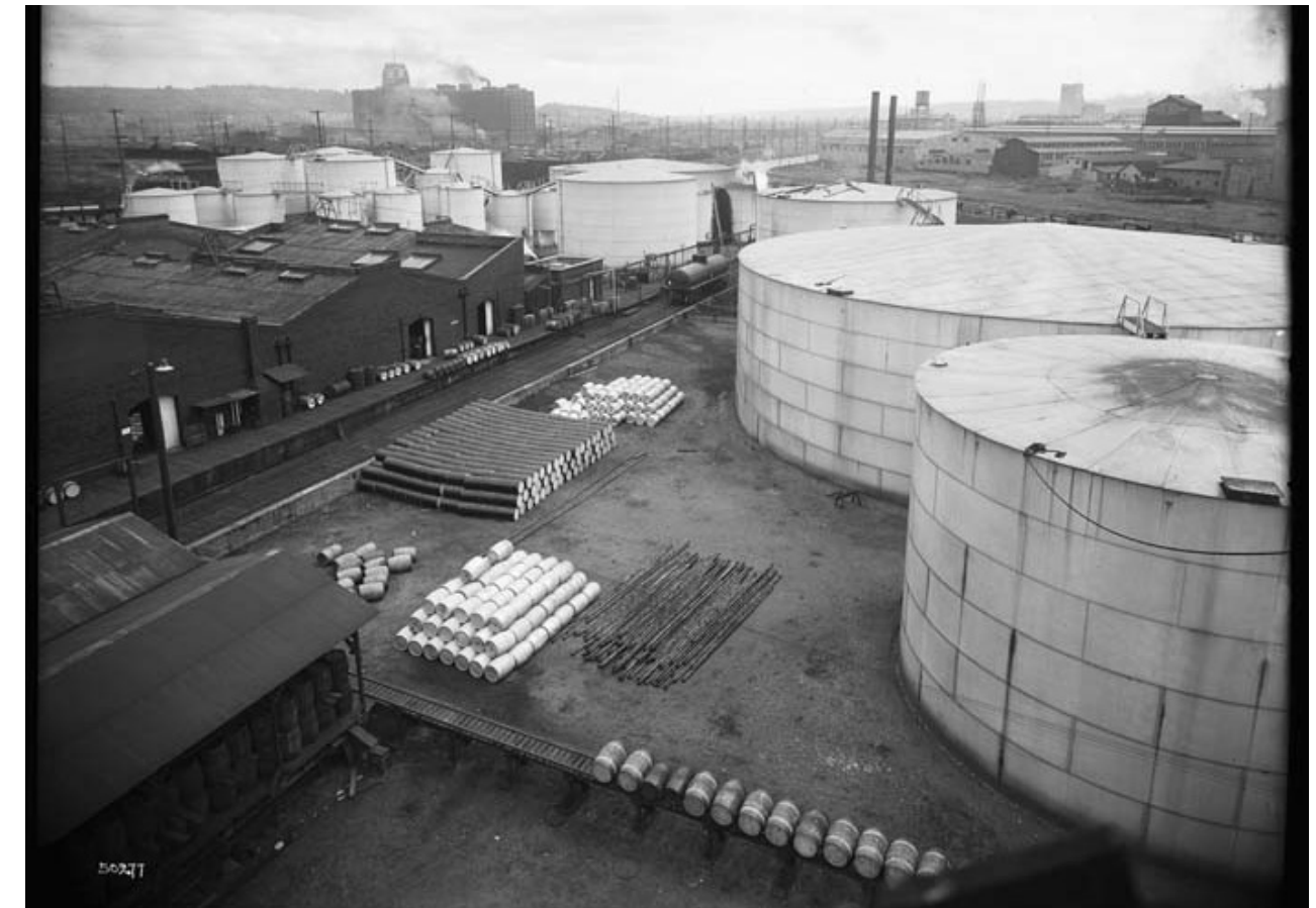
Figure 52: A typical Standard Oil facility on flat ground near the railroad, 1916. Image: Museum of History and Industry
