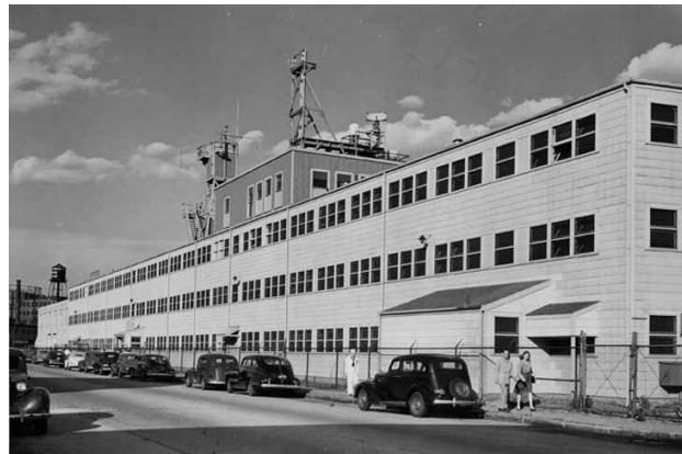
Figure 2: Building 20's regular geometric form and flexible wood structure made it ideal for a multitude of innovations. 1945. Image: http://webmuseum.mit.edu/detail.php?t=subjects&type=all&f=&s=Building+20&record=1
