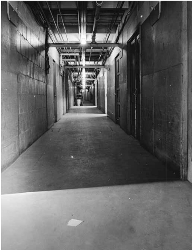
Figure 4: Exposed services inside MIT's Building 20, 1945. Image: http://webmuseum.mit.edu/detail.php?t=subjects&type=all&f=&s=Building+20&record=1
