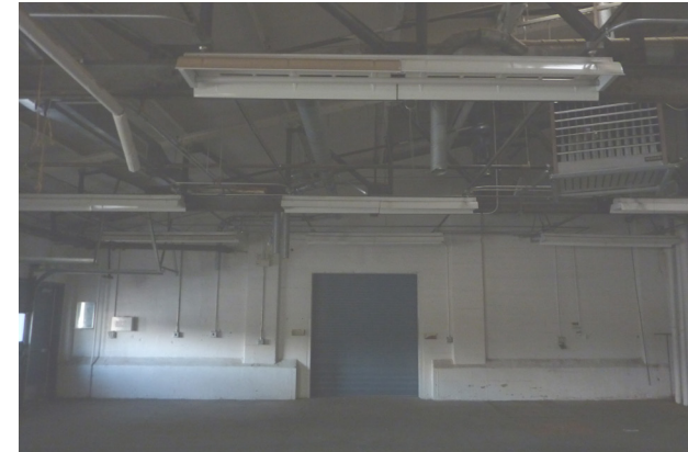
Figure 41: The interior of the east arm of the south building, 2013.
