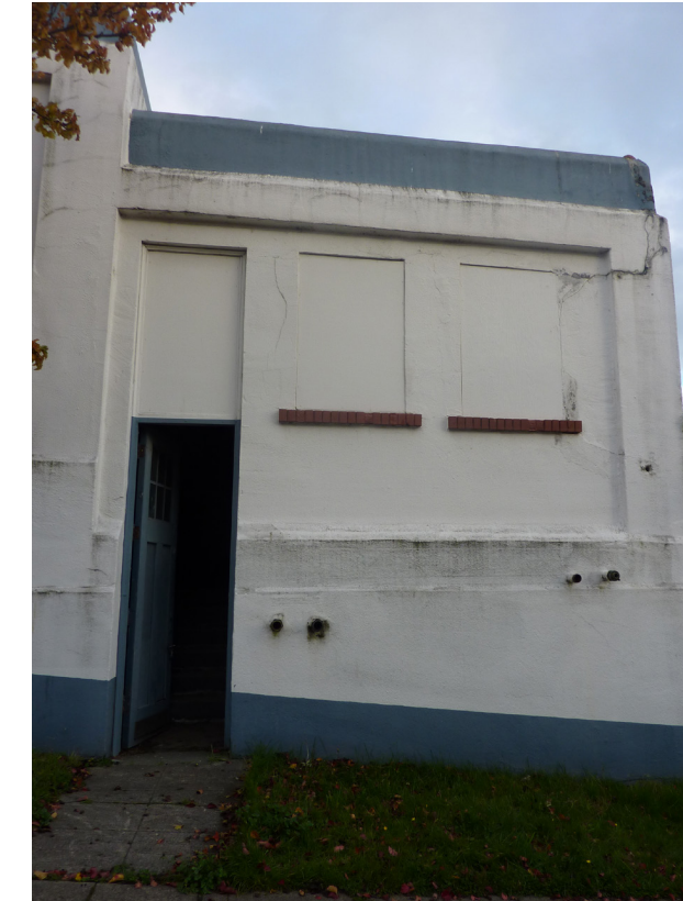
Figure 37: The entrance to the pump house along Woodlawn Avenue, 2013.
