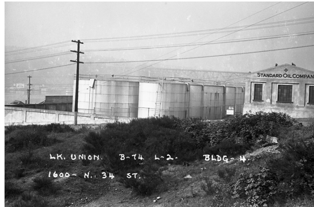
Figure 45: The fuel storage tanks originally occupied the central courtyard, 1937. Image: Washington State Archives, Puget Sound Regional Branch.
