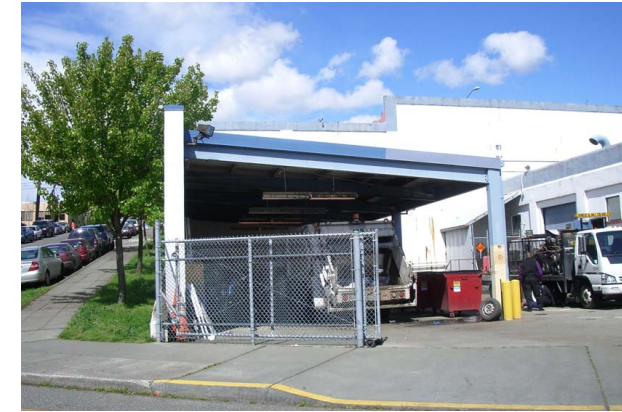
Figure 42: The carport was constructed in 1991 after the original structure was demolished. 2007. Image: Historic Landmark Nomination Form
