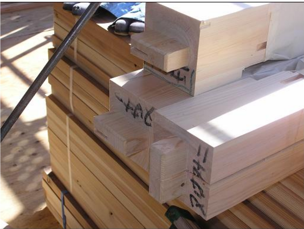
Picture 4. Power Builder uses pre-cut lumber. Those are sent to job sites from outside pre-cut factories. Power Builders do not have to store inventory at job sites.
