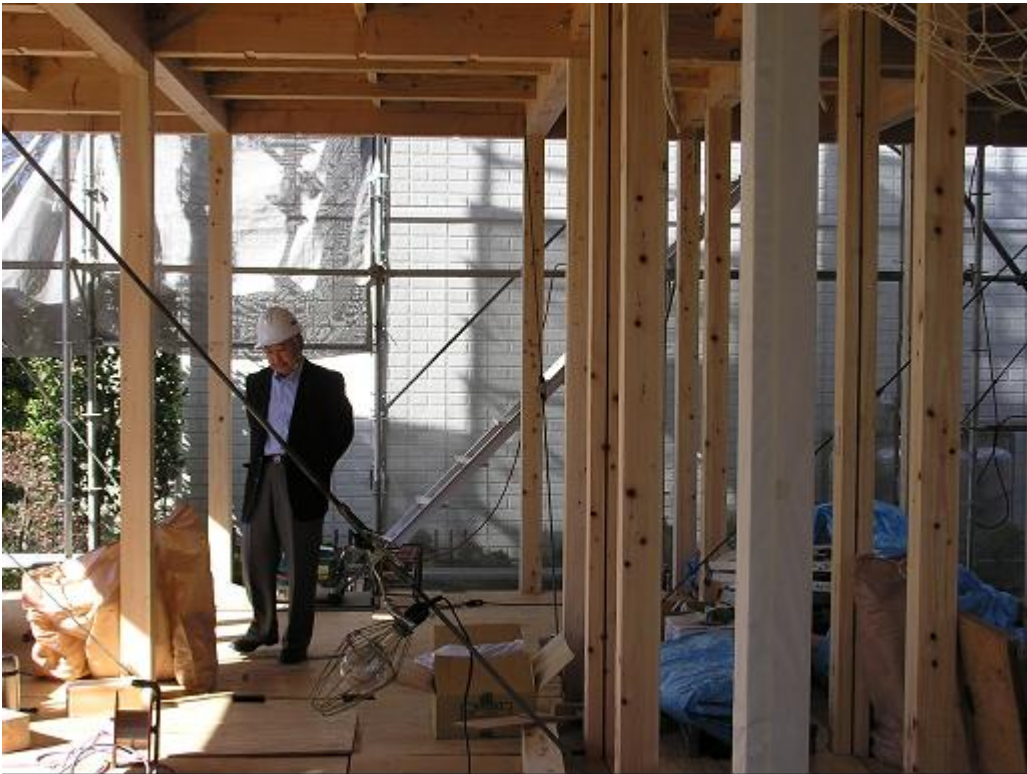
Picture 12. This self-proclaimed “power builder” utilizes hinoki for post and Douglas-fir for beam. However, they try to emphasize their “economy” aspect to attract price sensitive young generation.
