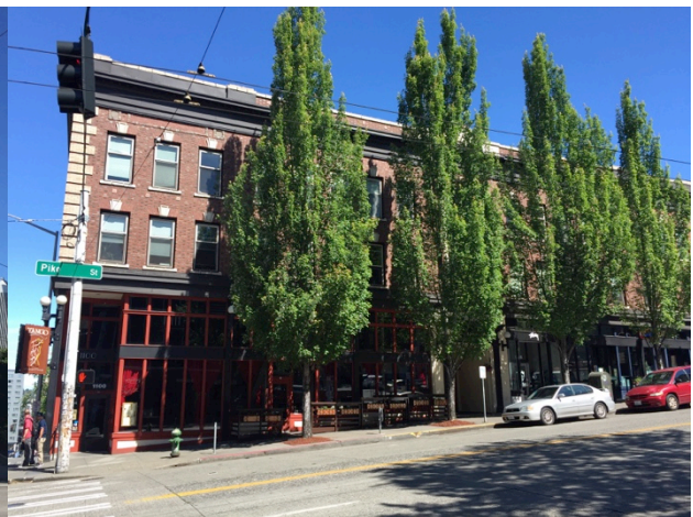
Figure 4-42 A2 Villa Apartments
