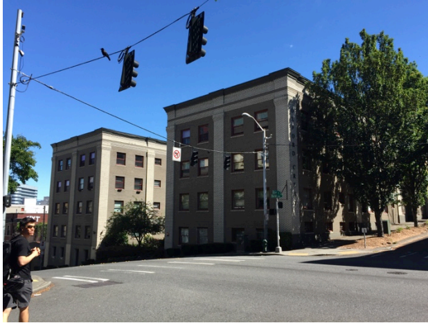
Figure 4-37 Oxford Crest Apartments
