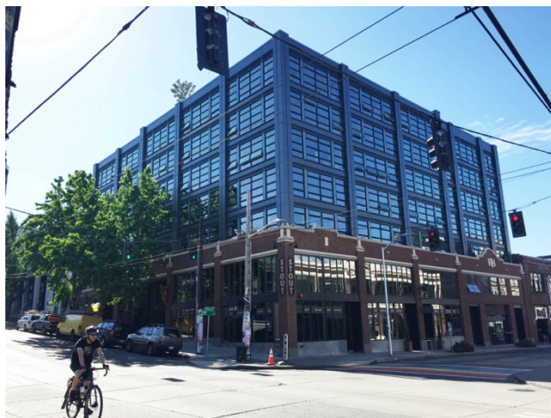
Figure 4-29 Sunset Electric Apartments
