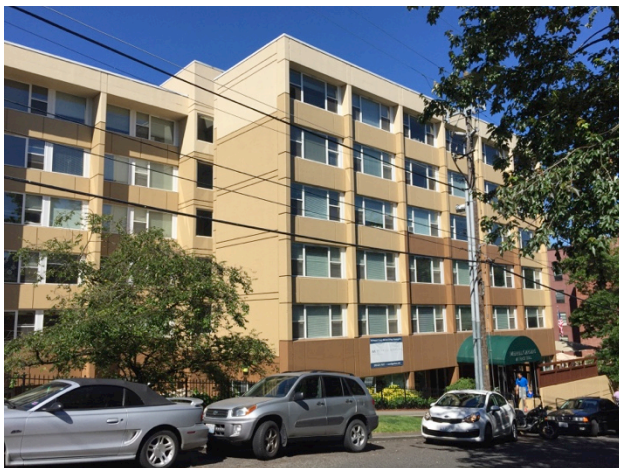
Figure 4-49 B5 Merrill Gardens at First Hill
