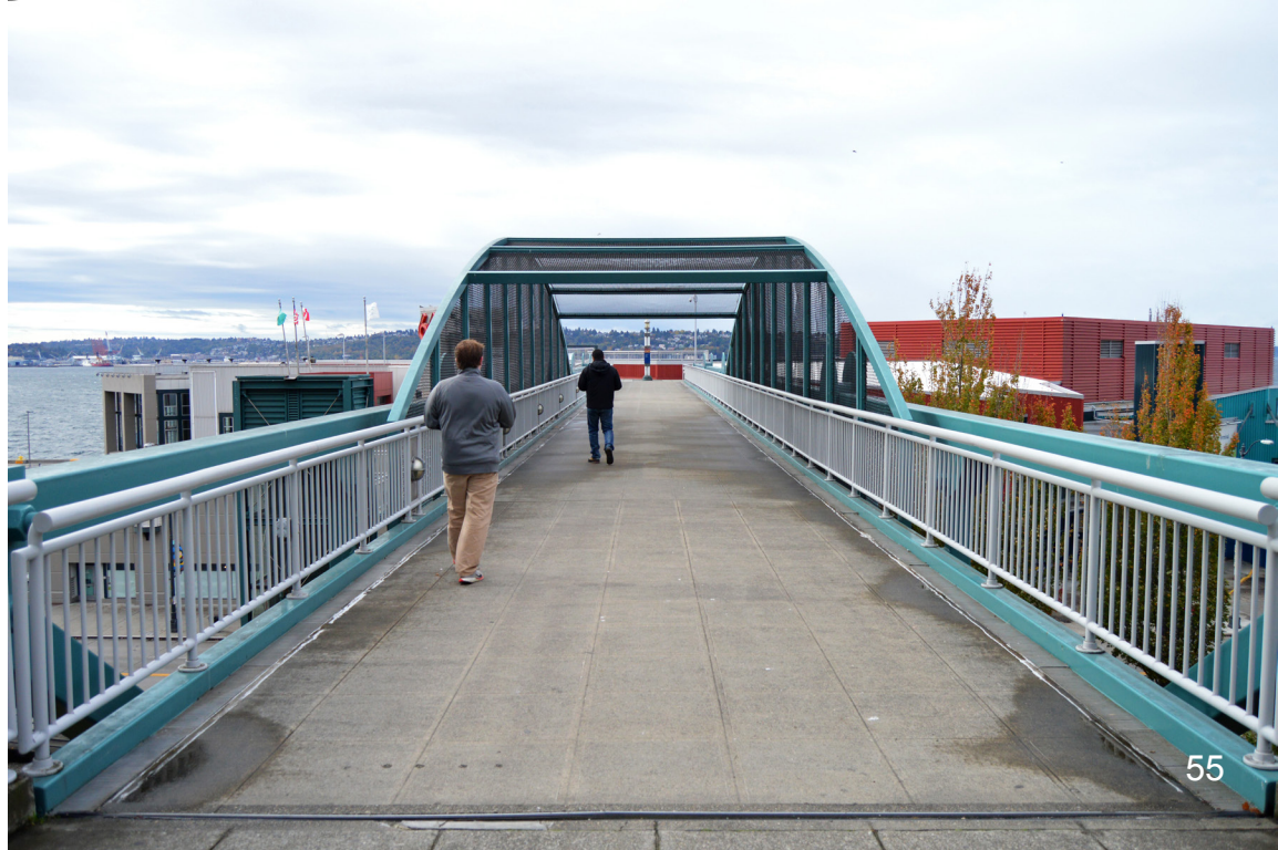
Figure 4.9 Photo of the Bell Street Bridge from the top of the bridge.
