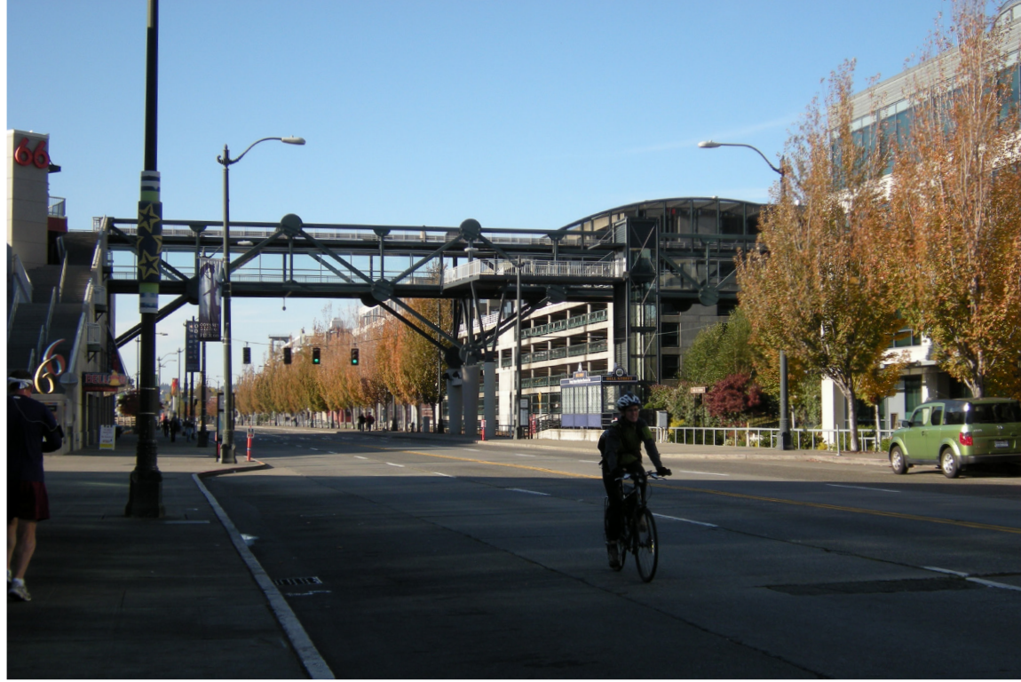
Figure 4.8 Photo of the Bell Street Bridge seen from the Alaskan Way.
