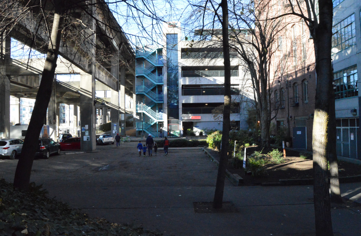
Figure 4.6 Site Photograph, Between the Alaskan Way Viaduct and the Fix/Madore Buildings
