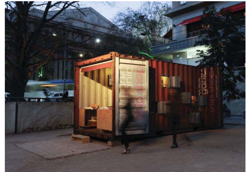
Fig: 4.4 Application of Freight Container System
