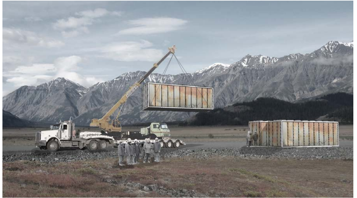
Fig: 8.19 Gallery Constructed on Site
