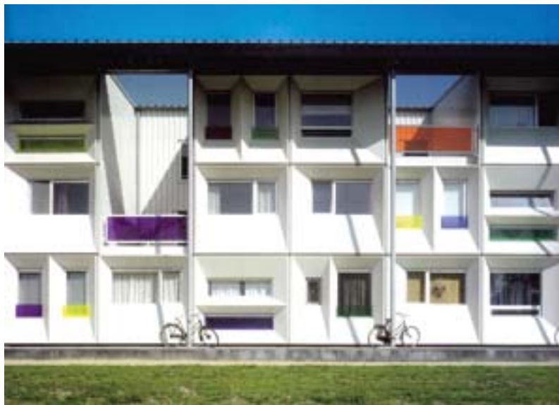
Fig: 4.6 Application of Building Container System
