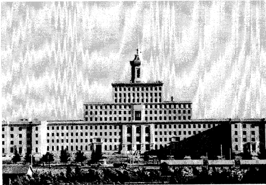
Figure 1.24: Central Broadcast Building, 1957
