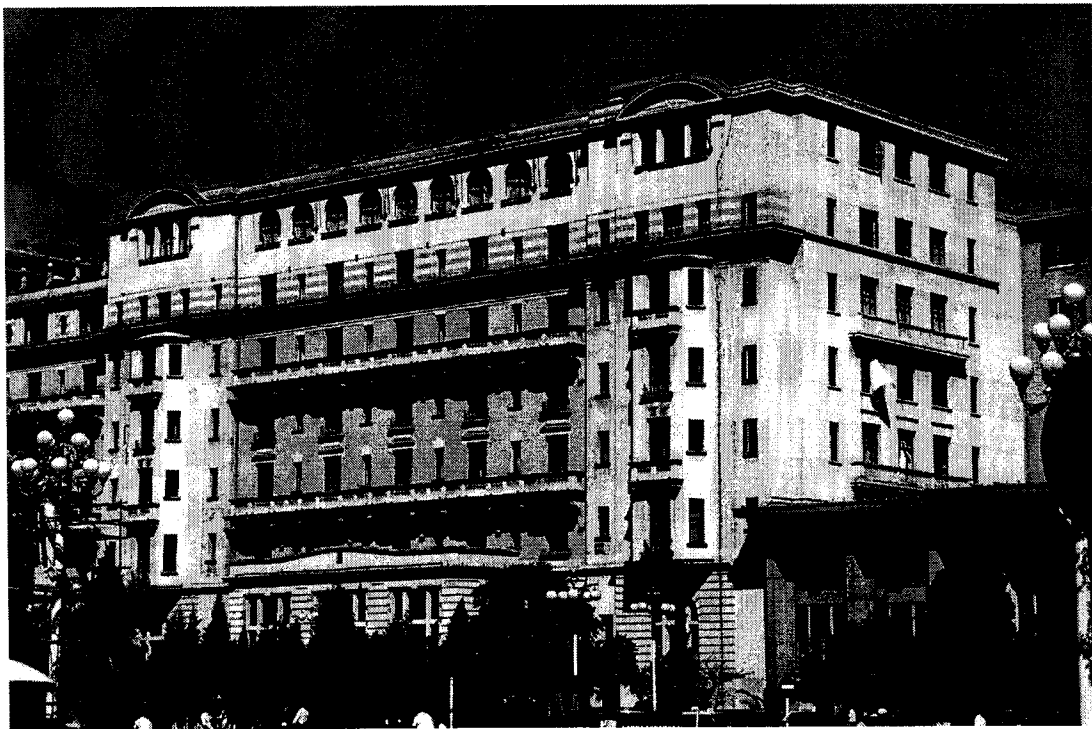
Figure 2.5: Beijing Hotel, Middle Building, 1917
