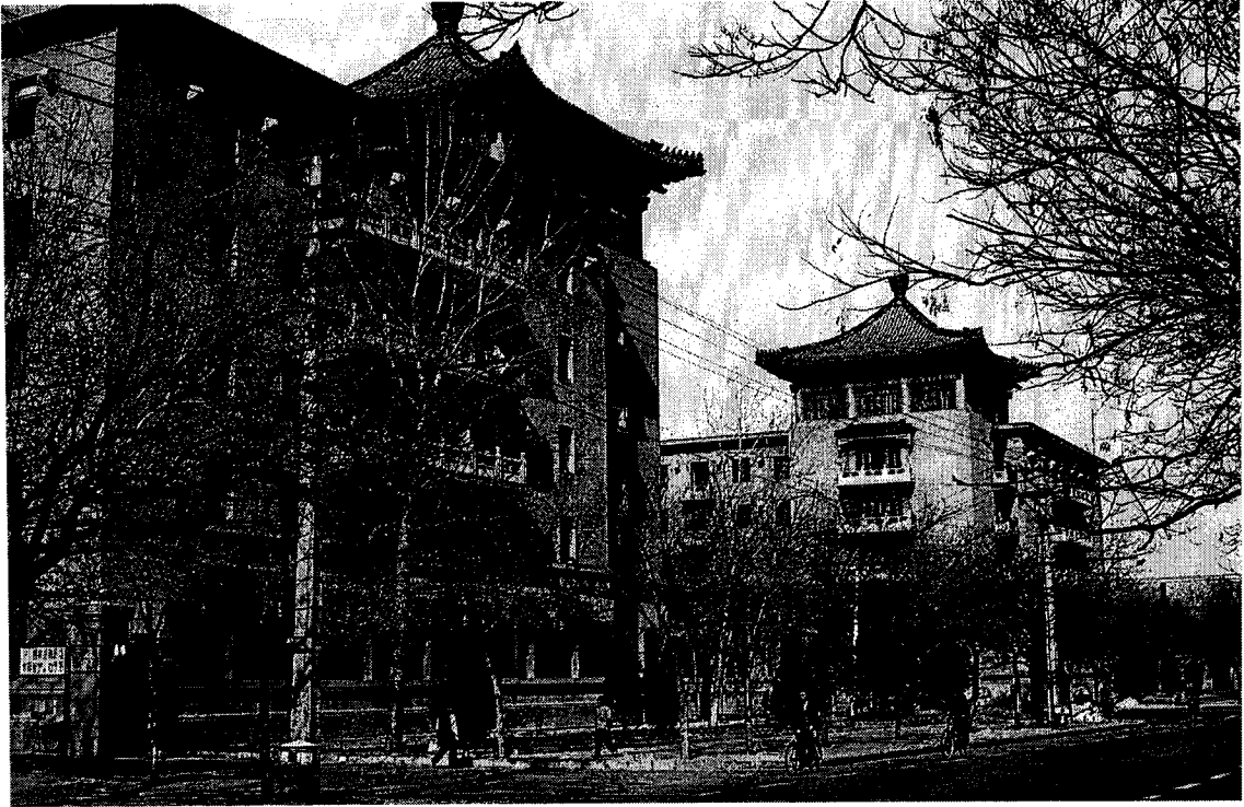
Figure 2.8: Sanlihe Office Buildings for Four Ministries and One Committee, 1954
