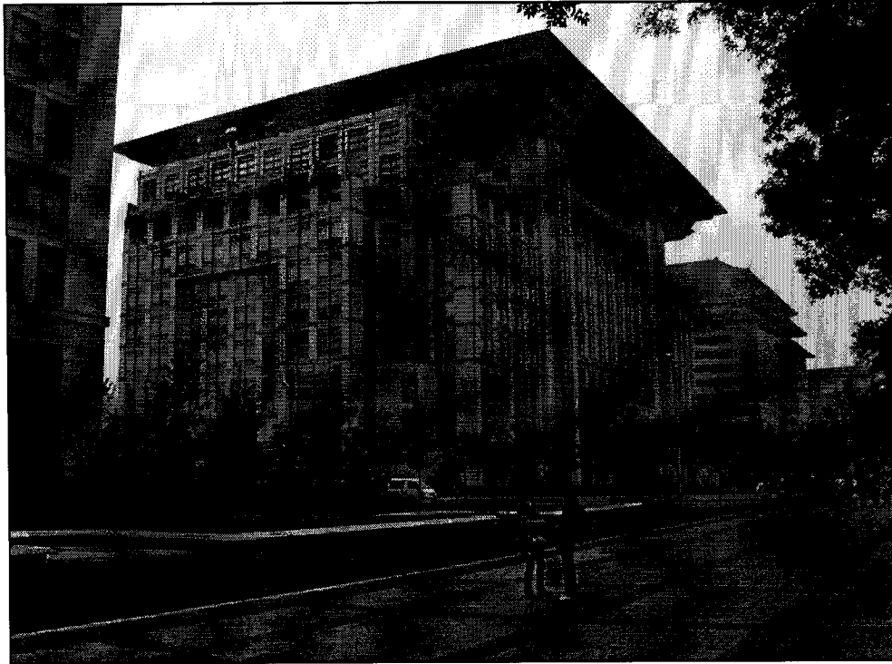
Figure 5.19: National Electricity Power Distribution Center, 1998
