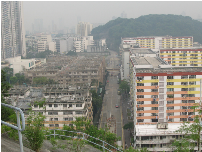
Fig.12 Demolished vs New Shek Kip Mei Estate taken by Nathan Tseng
