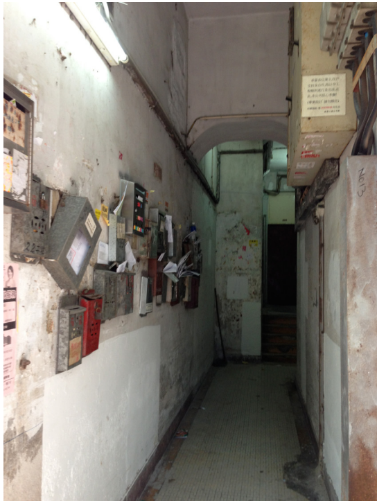
Fig. 40 Lack of security
