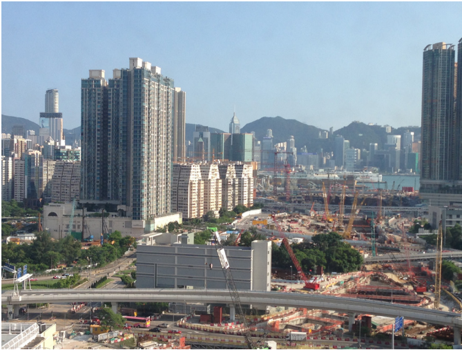
Fig. 38 Express Rail Link under construction
