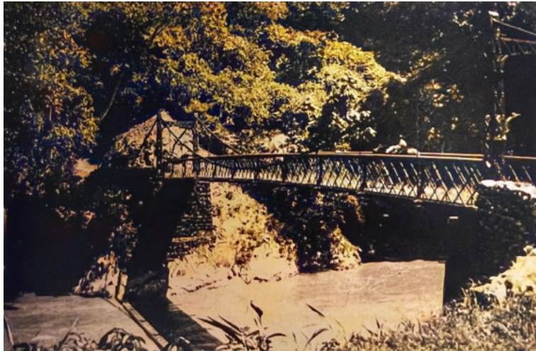
Figure A.3: British-constructed bridge across the Doyang river taken by Connie Shakespear, 1900-1902.
