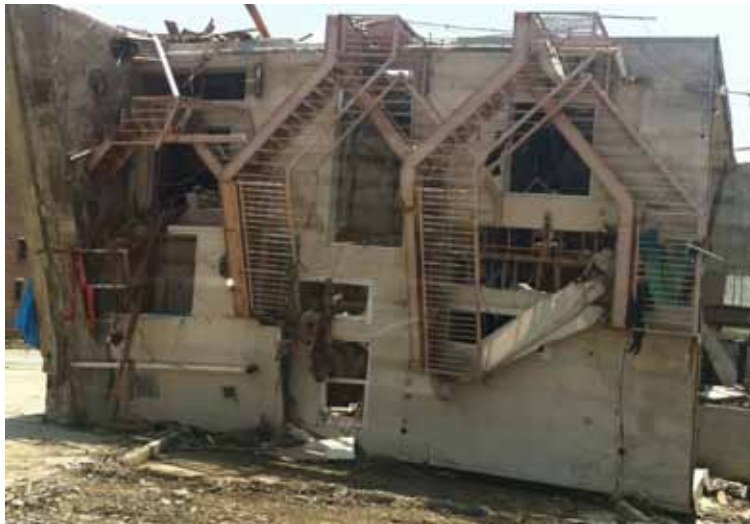
The tsunami toppled buildings from a combination of lateral force and liquefaction.
