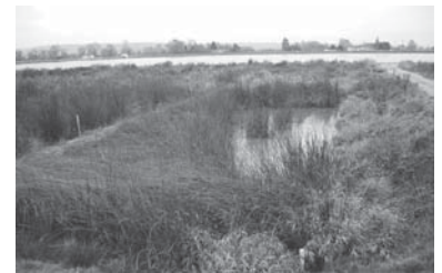
A pilot-scale constructed wetland at the city of Stanwood’s wastewater treatment facility, Snohomish County. Shown are two Scirpus acutus (bulrush) dominated marsh components, separated by a gravel berm.
